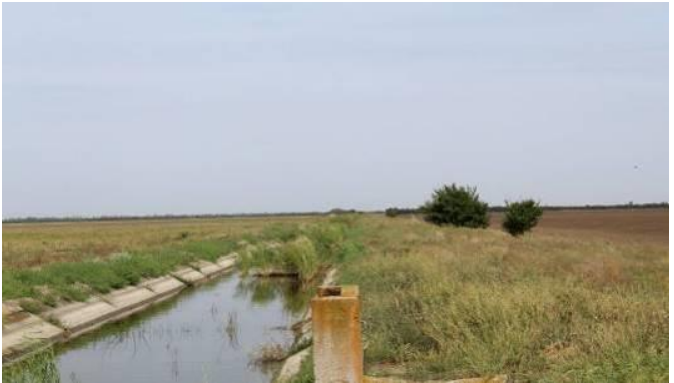
Fig. 4.9. Irrigation canal near the OHPL
