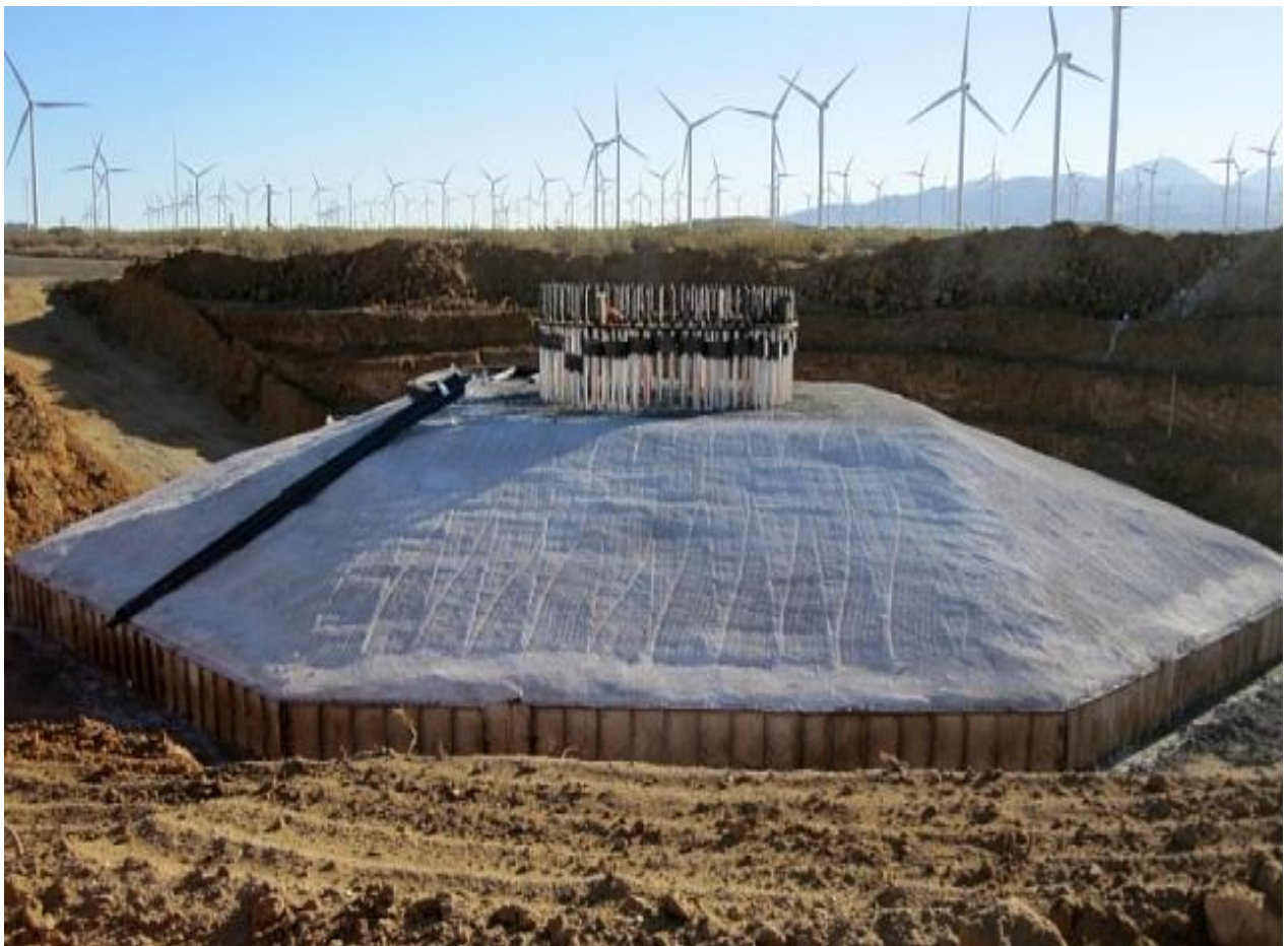
Fig. 4.92. The foundation of modern wind turbine generator
