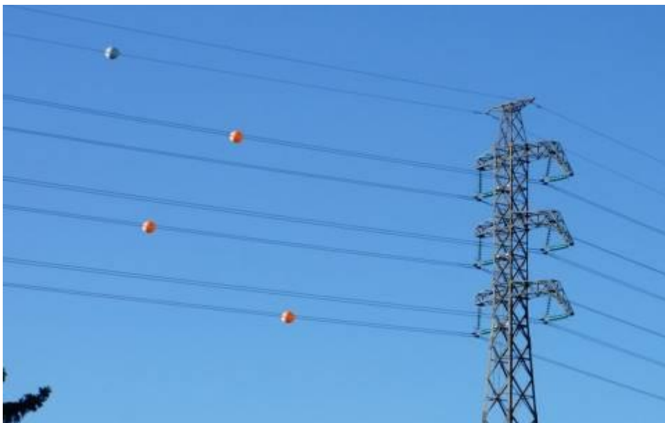
Fig. 4.50. Example of bullet-ball marker mounting on air-conductor wires
