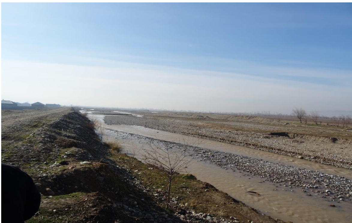
Photo 10 Existing embankment on the left bank
