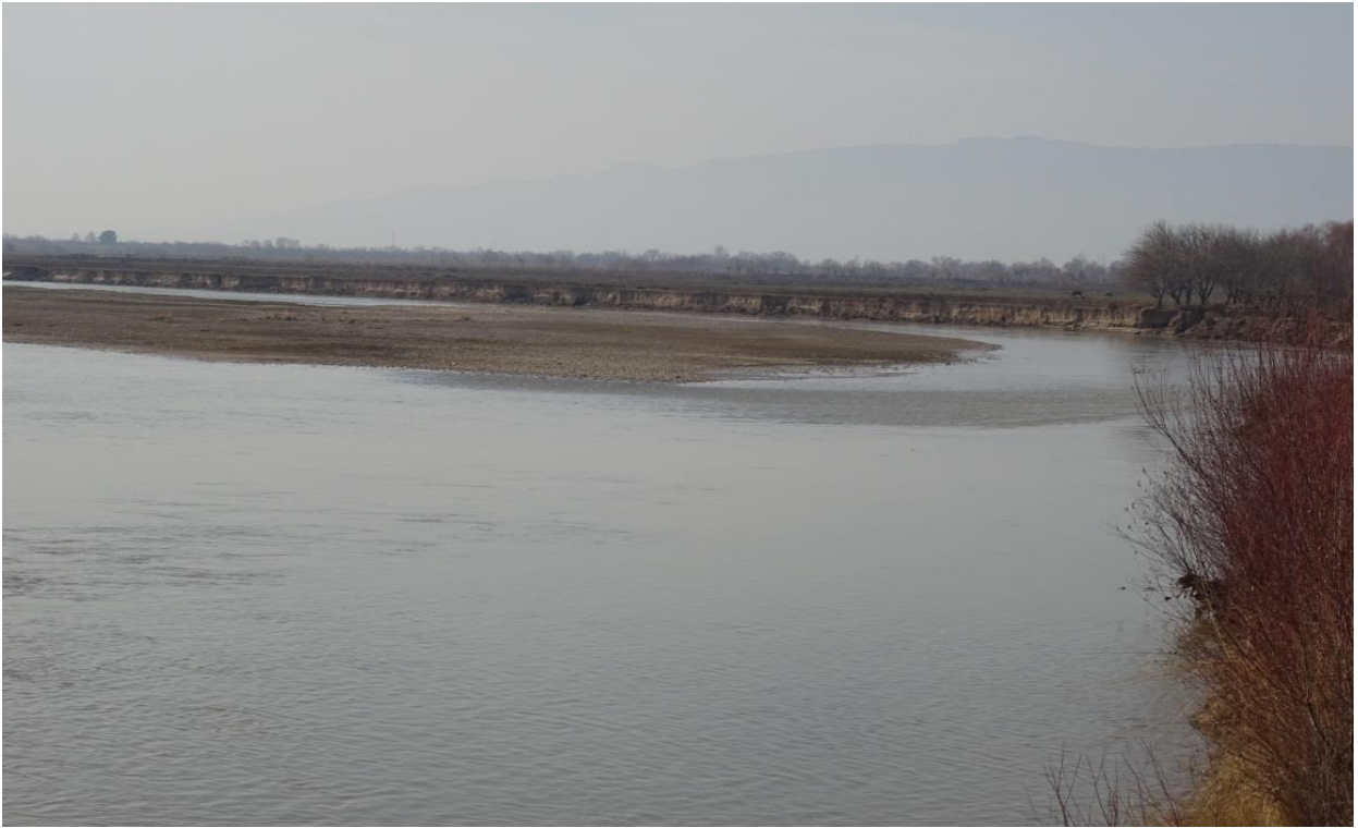
Photo 13 Damaged right bank of Kafernigan River
