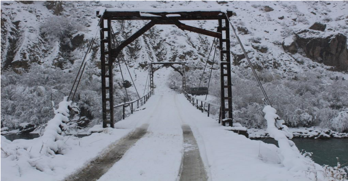
Photo 6 Bridge over river of Vanj on the road to Vanji bolo near the village of Chikhoh
