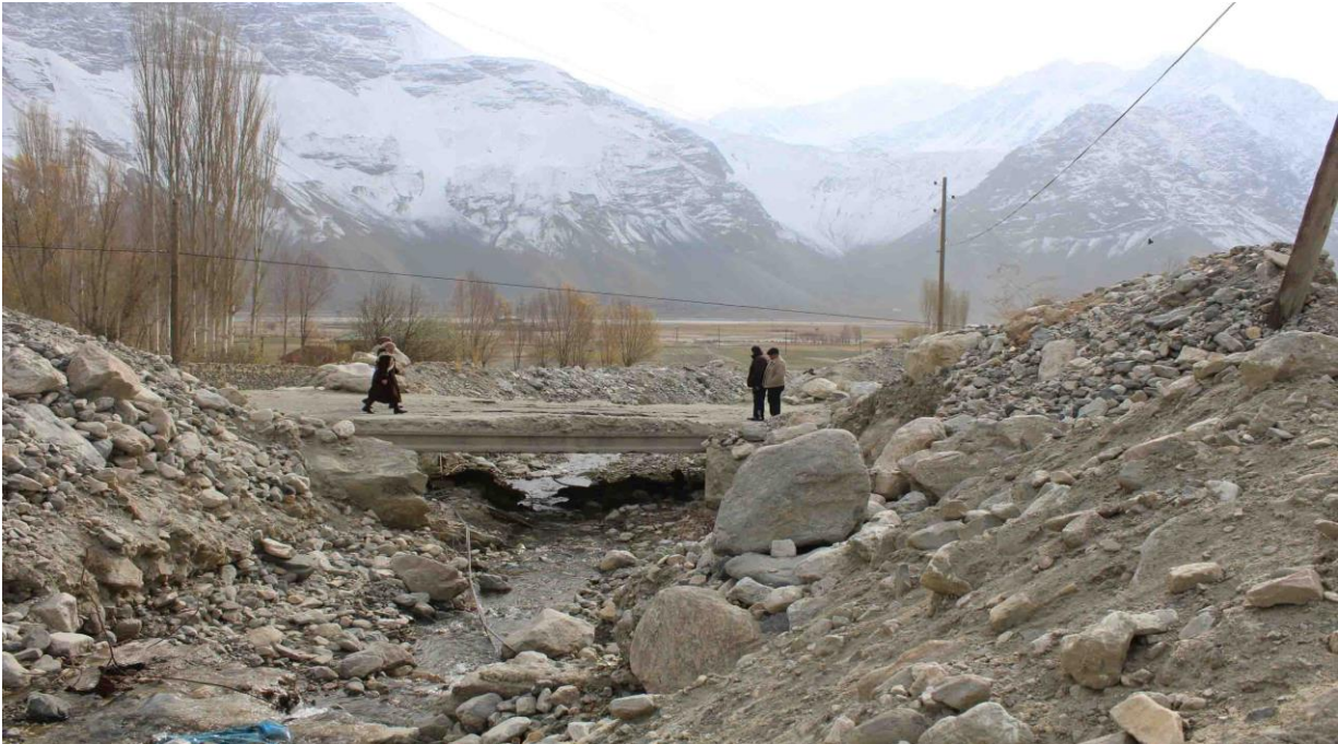
Photo 9 Bridge over Barushondara at km 538 of the road Dushanbe-Kulyab-Khorog-Kulma
