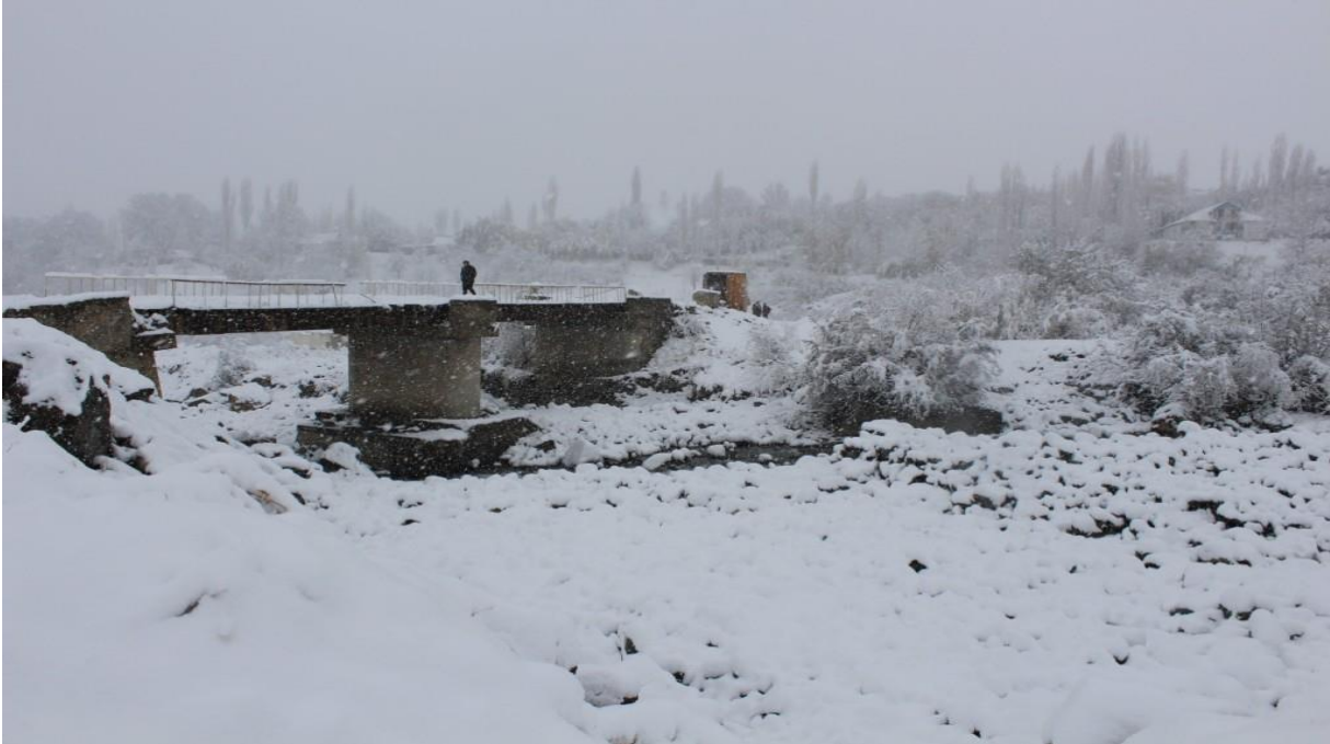
Photo 7 Bridge over the river of Obi-Sed on the road Vanji Bolo near the village of Sed
