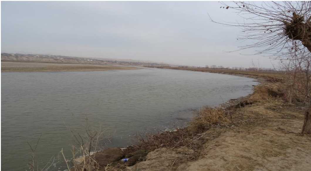
Photo 14 Flood No. 5 Hoshadi canal, Kafernigan River
