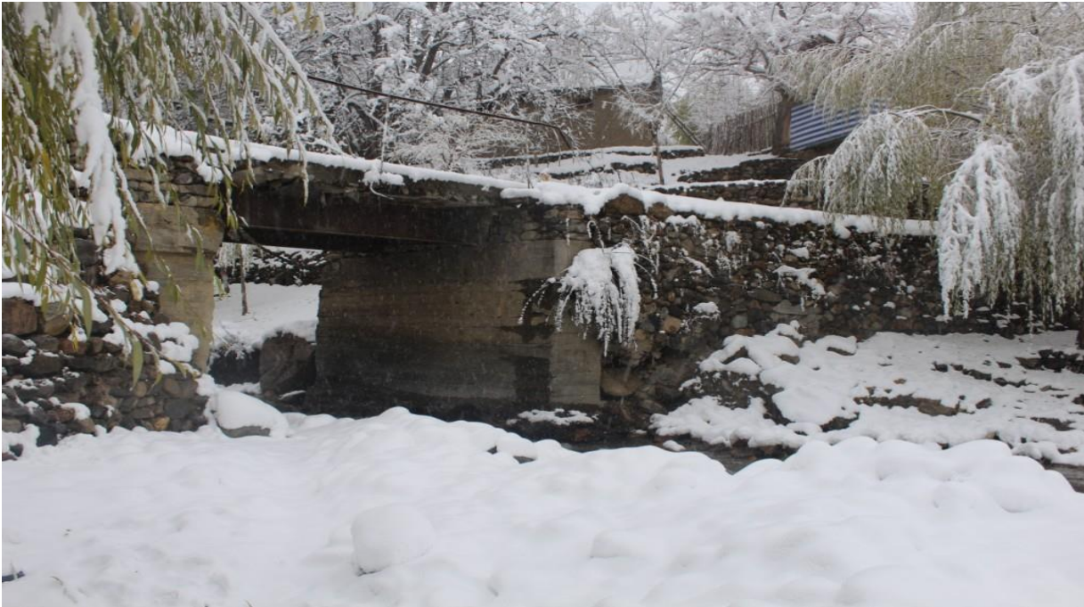
Photo 5 Bridge over the river Obi-Chikhoh on the road Chikhoh-Ravganda near the village Chikhoh of Vanj district
