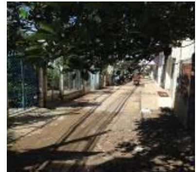
Degraded concrete alley
