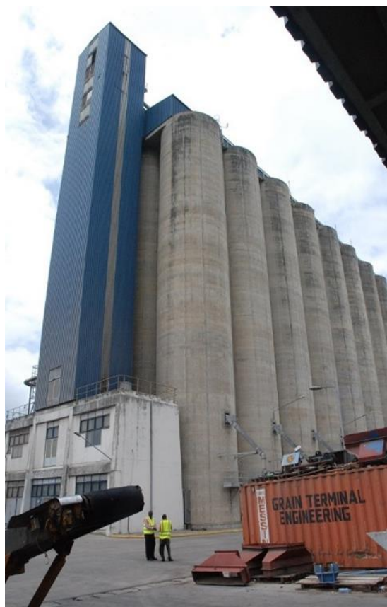
Figure 4-8 TPA grain silos close to Bandari Road. Not in use due to poor condition of the installations.
