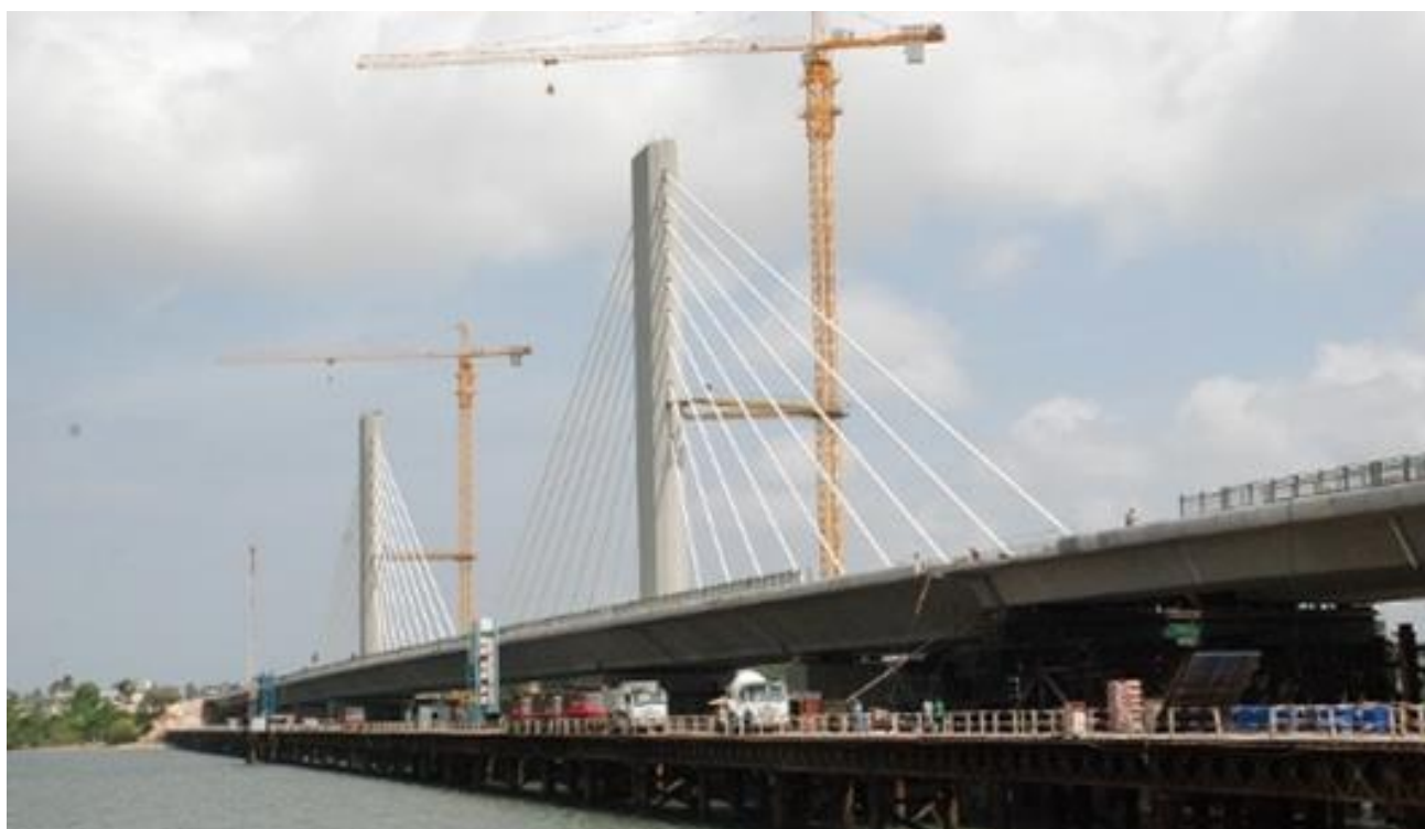
Figure 4-25 Kigamboni Bridge under construction (January 2016).
