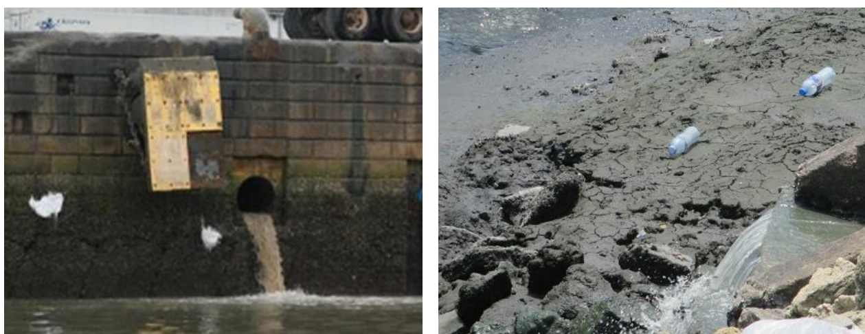
Figure 4-11 Portion of Berth 3 (left) showing gravity block structure and one of several storm water drains discharging dirty water into the Port, on a day of heavy rainfall (15 December 2015). There is concern that on days of heavy rainfall, spilt fertiliser from around the mid port shed also gets swept into the drains and discharged to sea. One of six drain discharging into the channel of the lower Gerezani Creek (on a non-rainy day), close to Malindi Wharf (right).
