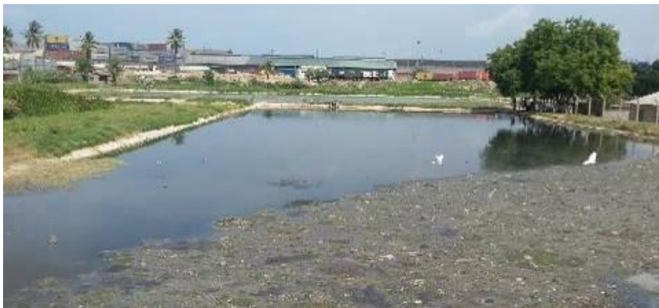
Figure 4-10 Part of the Kurasini oxidation ponds used by TPA for disposal of liquid waste.
