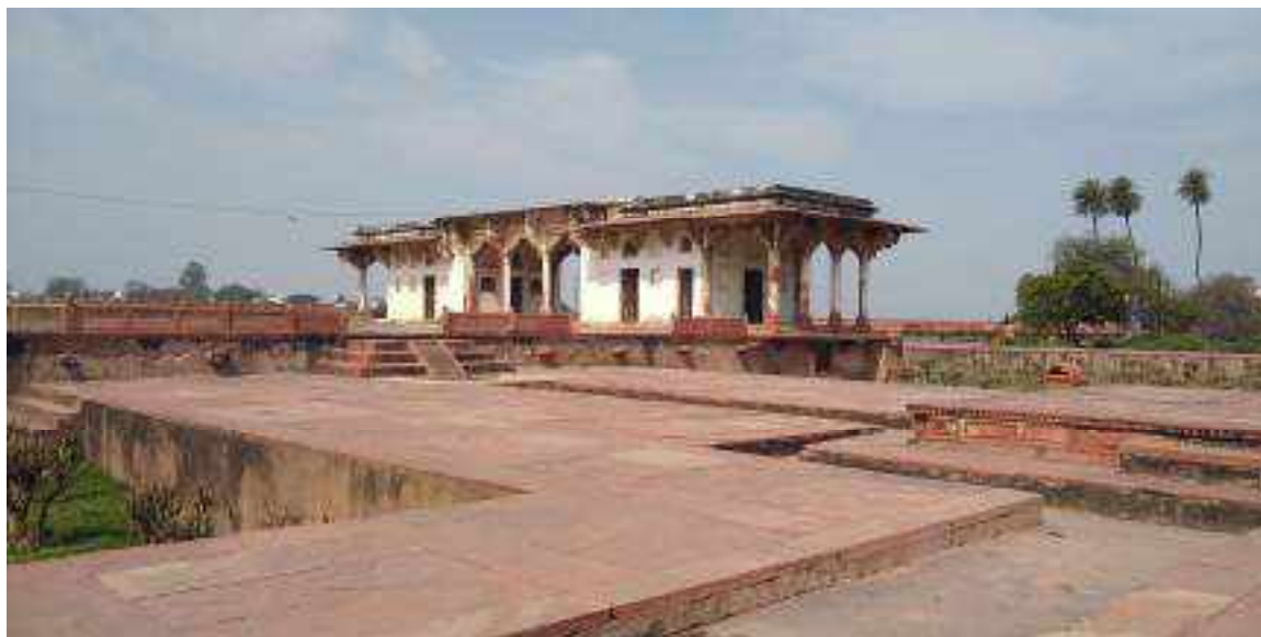
Image showing Ram Bagh houses and terraces
