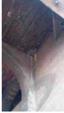
Figure 55: Moisture ingress
