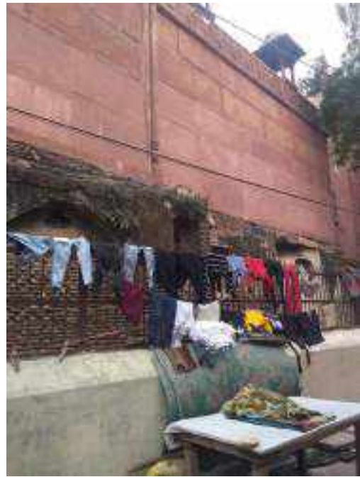
The rear view of the mosque there used to be a larger platform which does not existing anymore.
