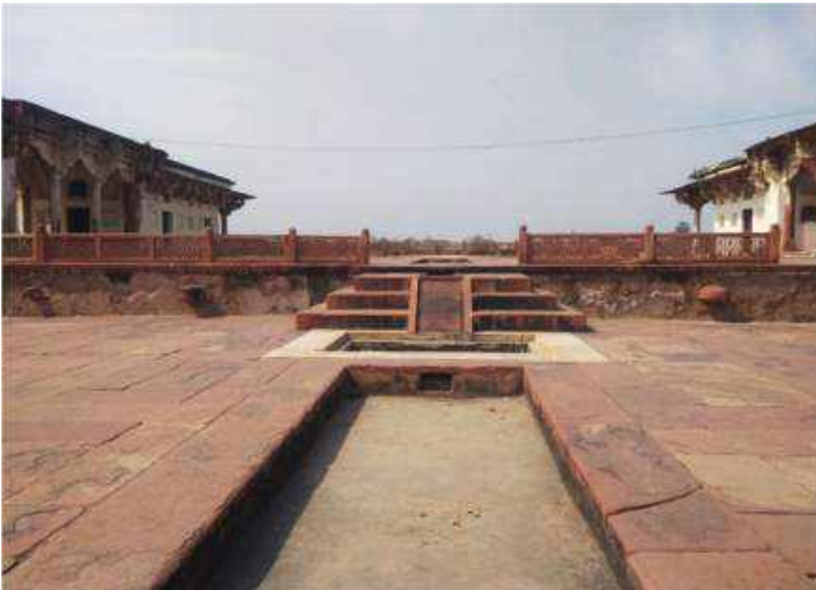
Condition of terraces of charbagh are stable. Signal storey houses are also in stable condition. There are signs of stone deterioration.
