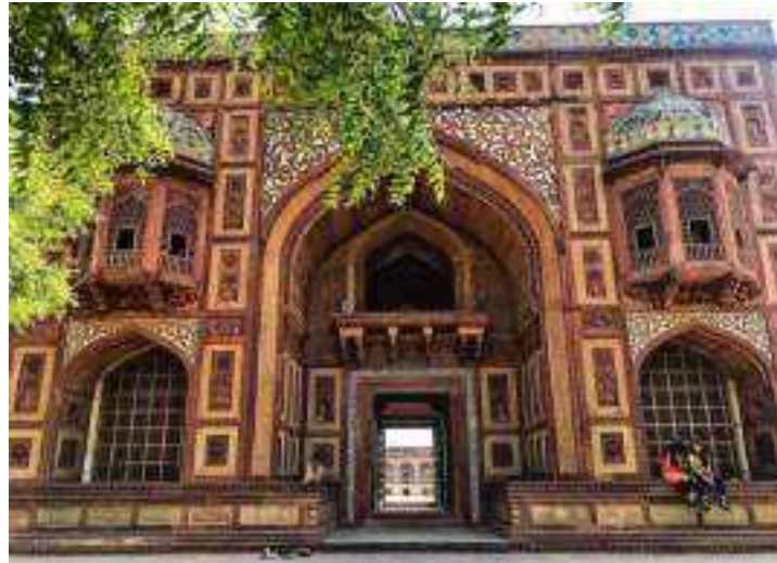
Image.5.2.5 North view of Kanch Mahal
