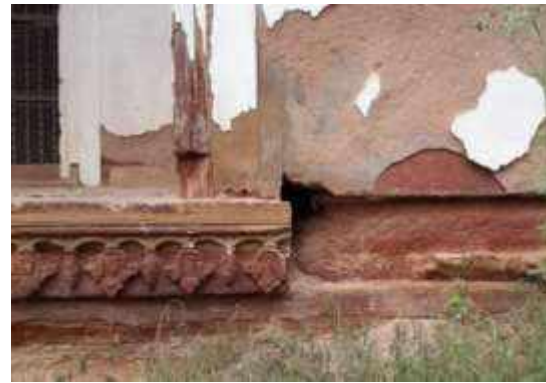
Figure 52: Openings at Base
