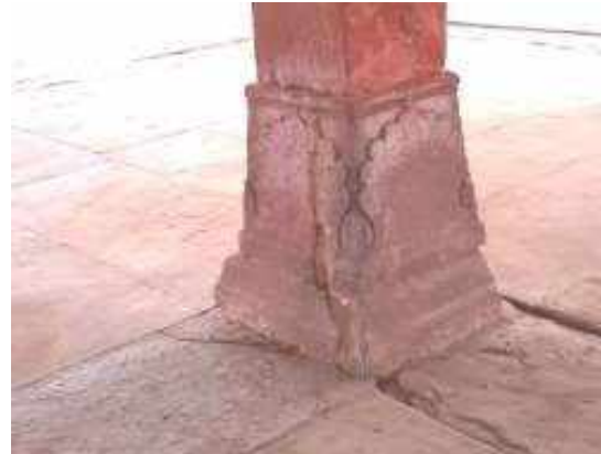
Figure 47: Wind Erosion
