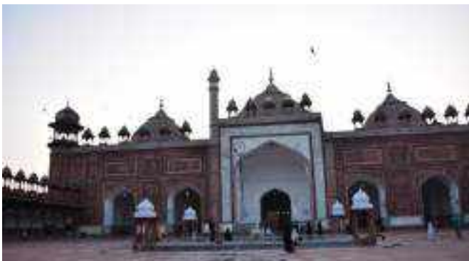
Image 5.2.14 External view of Jama Masjid bays from internal courtyard
