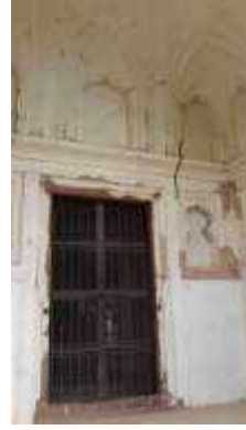
Figure 49: Vertical Crack
