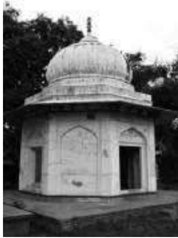
Plaster cracks on exterior surface
