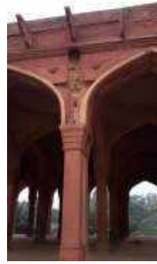
Figure 44: Vertical Crack
