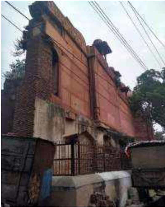
The view of mosque from north west direction showing a brick masonry supporting the mosque from further collapse
