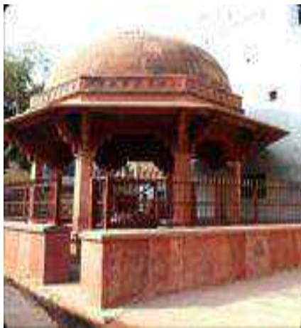
Image 5.2.12 External view of Barah Khamba
