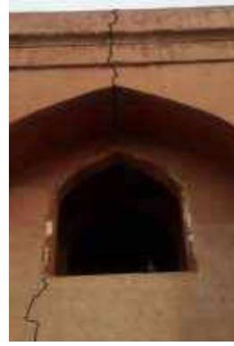
Figure 30: Vertical Crack
