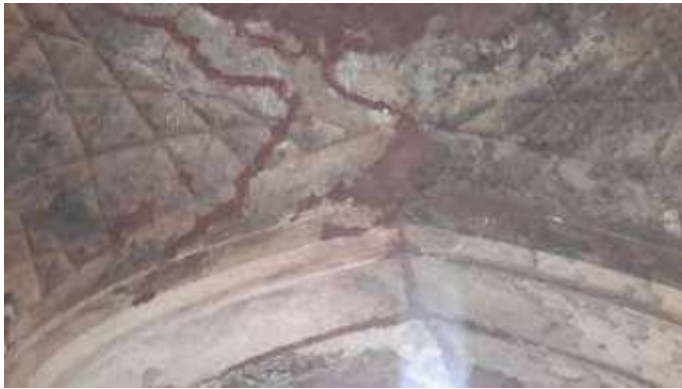
Figure 27 Cracks in the ceiling
