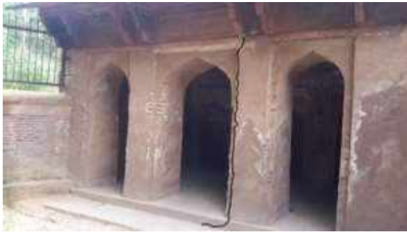
Figure 41: Vertical cracks
