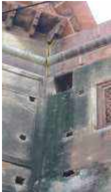
Figure 60: Vertical Crack
