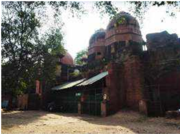
The view Shahi Lal mosque from north east direction which got partly collapsed. As the mosque is in use, temporary shed has been added at entry
