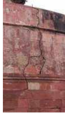
Figure 22: Vertical Crack
