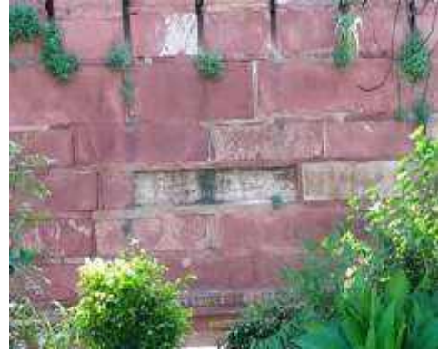
Figure 23: Loss of Cladding
