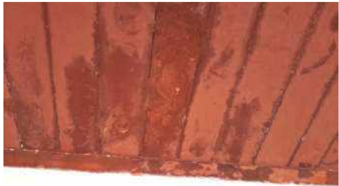
Figure 62: Water Ingress in roof
