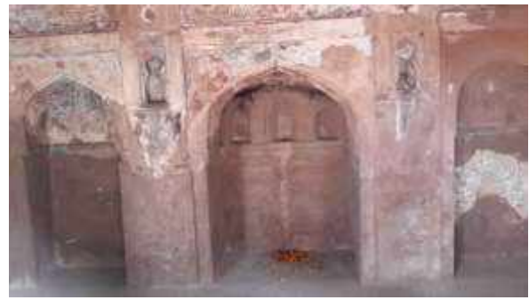
Figure 42: Plaster Delamination
