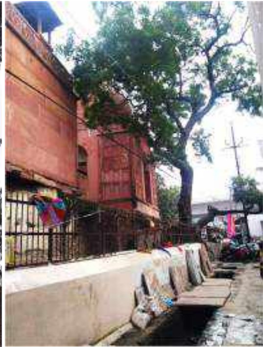
The rear view of the tomb with drainage nala along boundary wall
