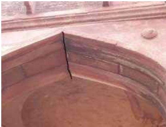
Figure 46: Structural Crack
