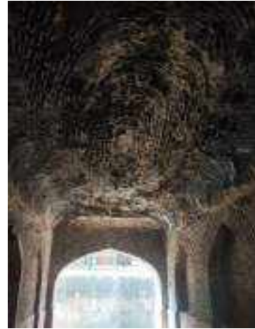
Exposed ceiling masonry of platform of the tomb
