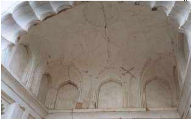
Figure 51: Structural Crack
