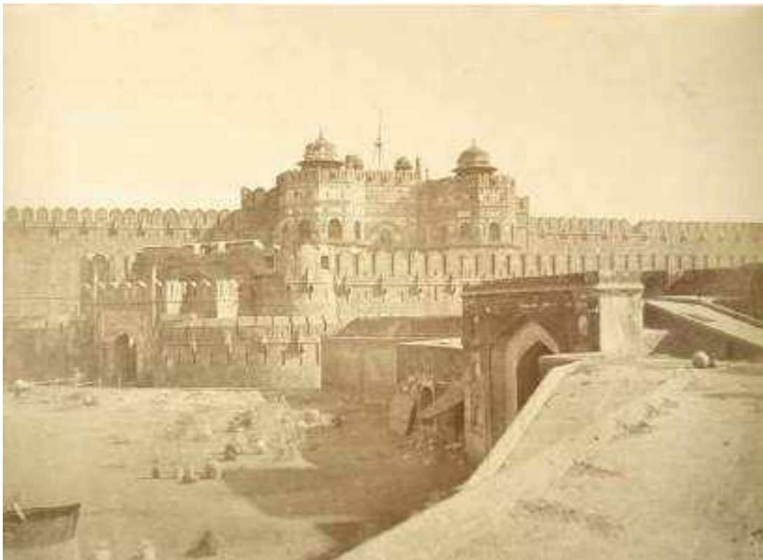
Image 20 A view of Delhi gate taken from the south west, Agra fort, Agra, Source: British Library Collection
