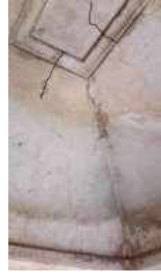
Figure 50: Horizontal Crack
