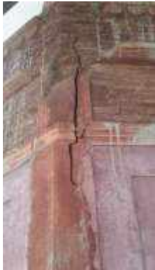
Figure 36: Vertical Crack
