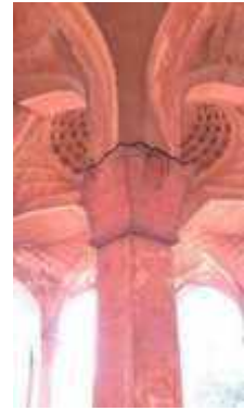
Figure 45: Horizontal Crack
