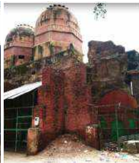
The image showing collapsed third dome of the mosque and temporary supports of brick masonry.
