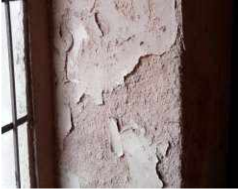
Figure 57: Plaster removal
