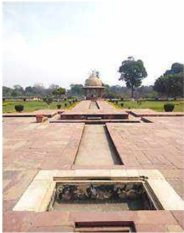
Condition of terraces are stable. There are signs of stone deterioration in patches all over.
