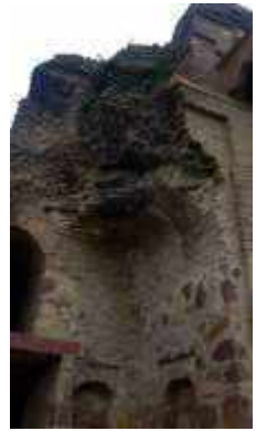
Figure 28: Vegetation Growth and structural damage
