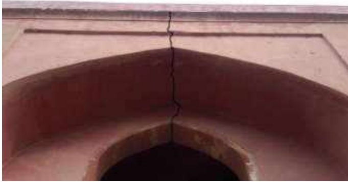
Figure 32: Structural crack
