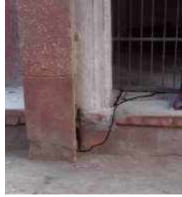
Figure 56: Horizontal Crack
