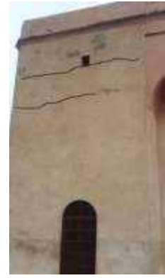
Figure 31: horizontal crack
