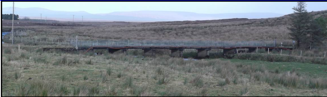
Plate 17-29: Site CH-16 – Srahnakilly - Bridge
