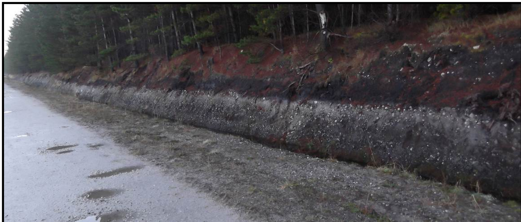
Plate 17-39: Exposed Edge to Internal Access Road showing peat overlying gravelly sandy subsoils
