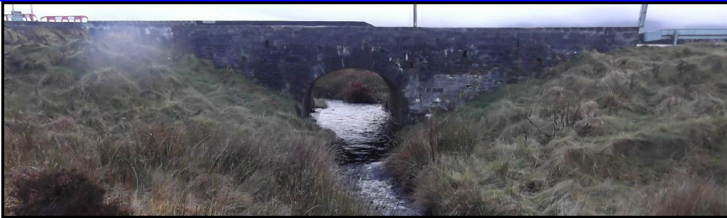
Plate 17-36: Site CH-22 – Moneynierin – Road Bridge
