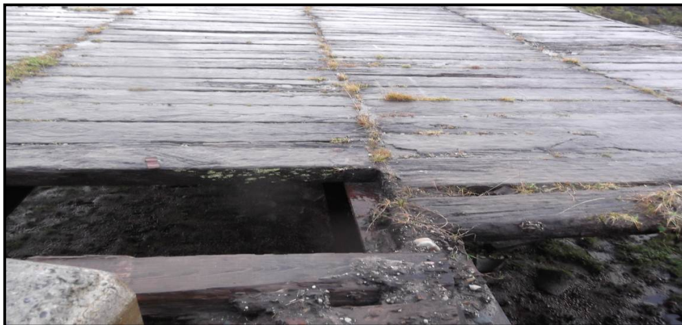
Plate 17-32: Site CH-19 – Detail to surface of railway bridge
