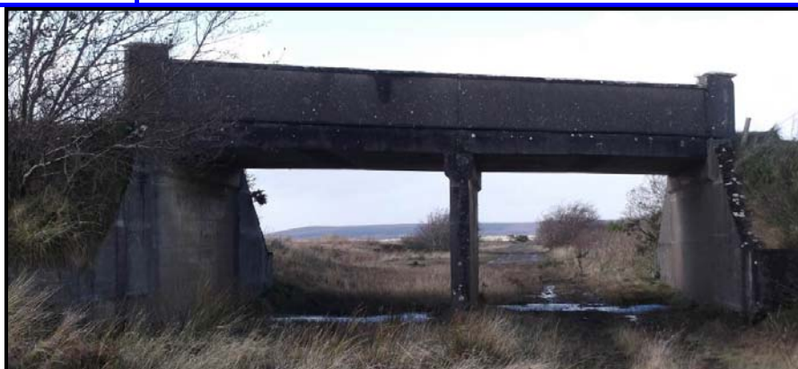
Plate 17-30: Site CH-17 - Srahnakilly - Road Bridge
