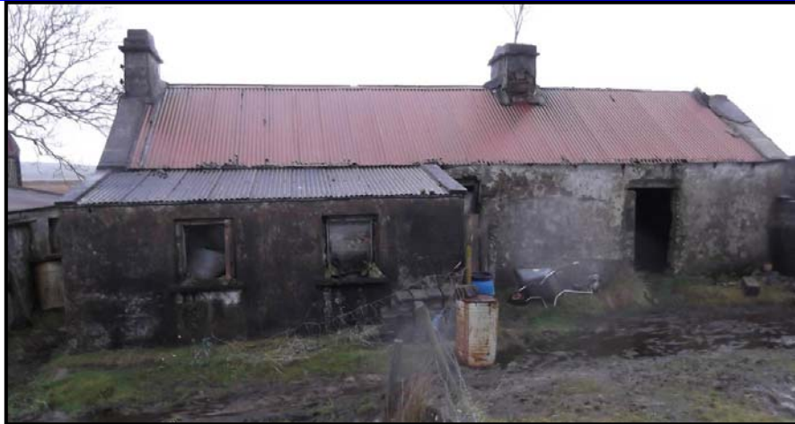
Plate 17-25: Site CH-12 - Cottage
