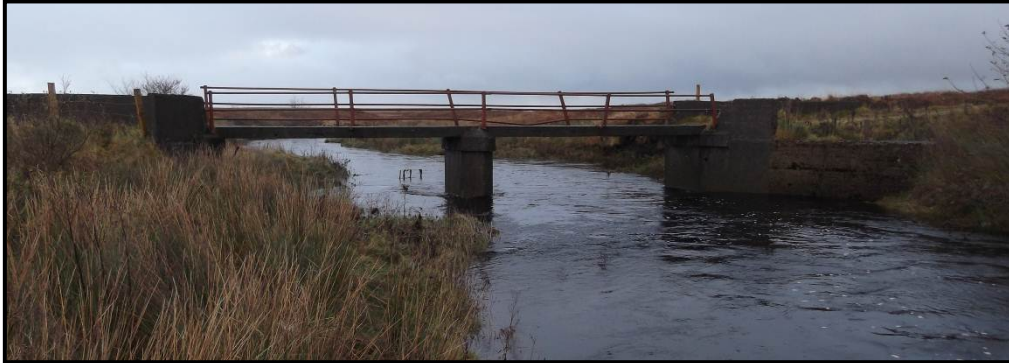
Plate 17-27: Site CH-14 - Srahnakilly - Bridge
