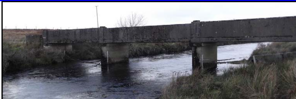
Plate 17-28: Site CH-15 - Srahnakilly – Bord na Móna Bridge
