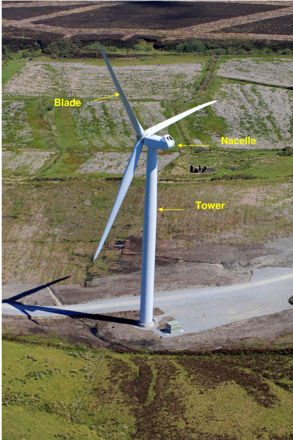
Figure 2-2: Typical turbine components ( ESB Curryfree wind farm )
