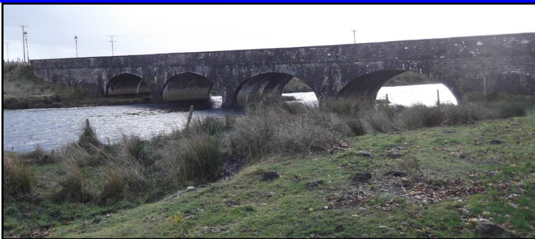
Plate 17-33: Site CH-19 – Bellacorick Bridge
