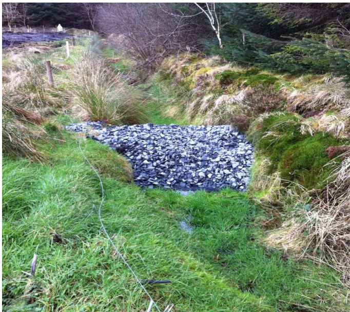
Plate 19-3: Typical stone check dam in a drainage ditch
