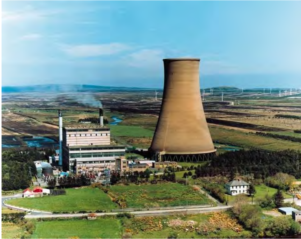
Plate 2-1: Bellacorick power station
