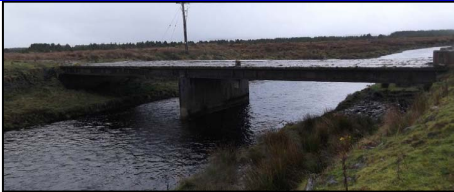
Plate 17-31: Site CH-18 – Srahnakilly – Railway Bridge
