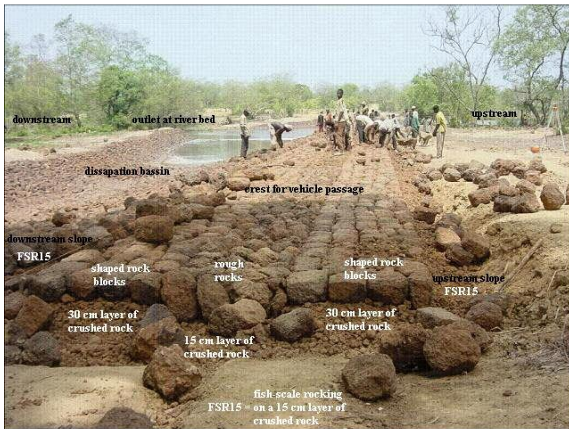
Figure 5: Details of the Labor-Intensive Fish-Scale Rocking System Utilizing Laterite or Granite Rock
