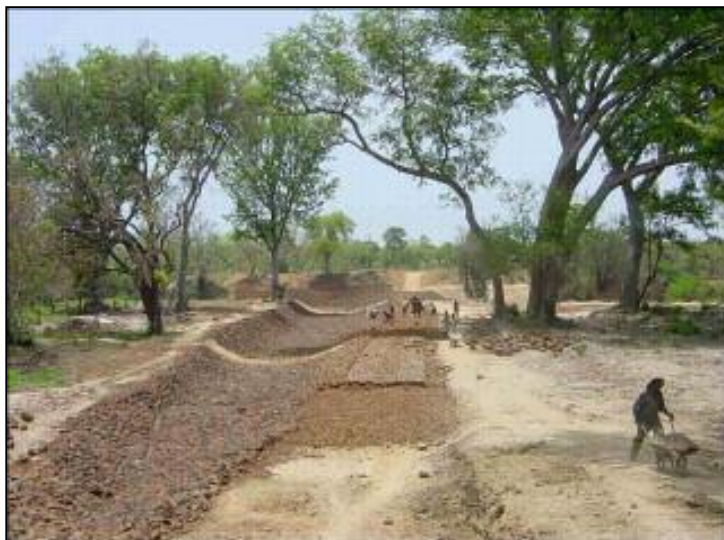
Figure 6: Construction of a 180 m long spillway dike on the Sissili River at Naguio, Nazinga Game Ranch, using labour-intensive methods and locally-available materials that incorporate a dissipation basin
