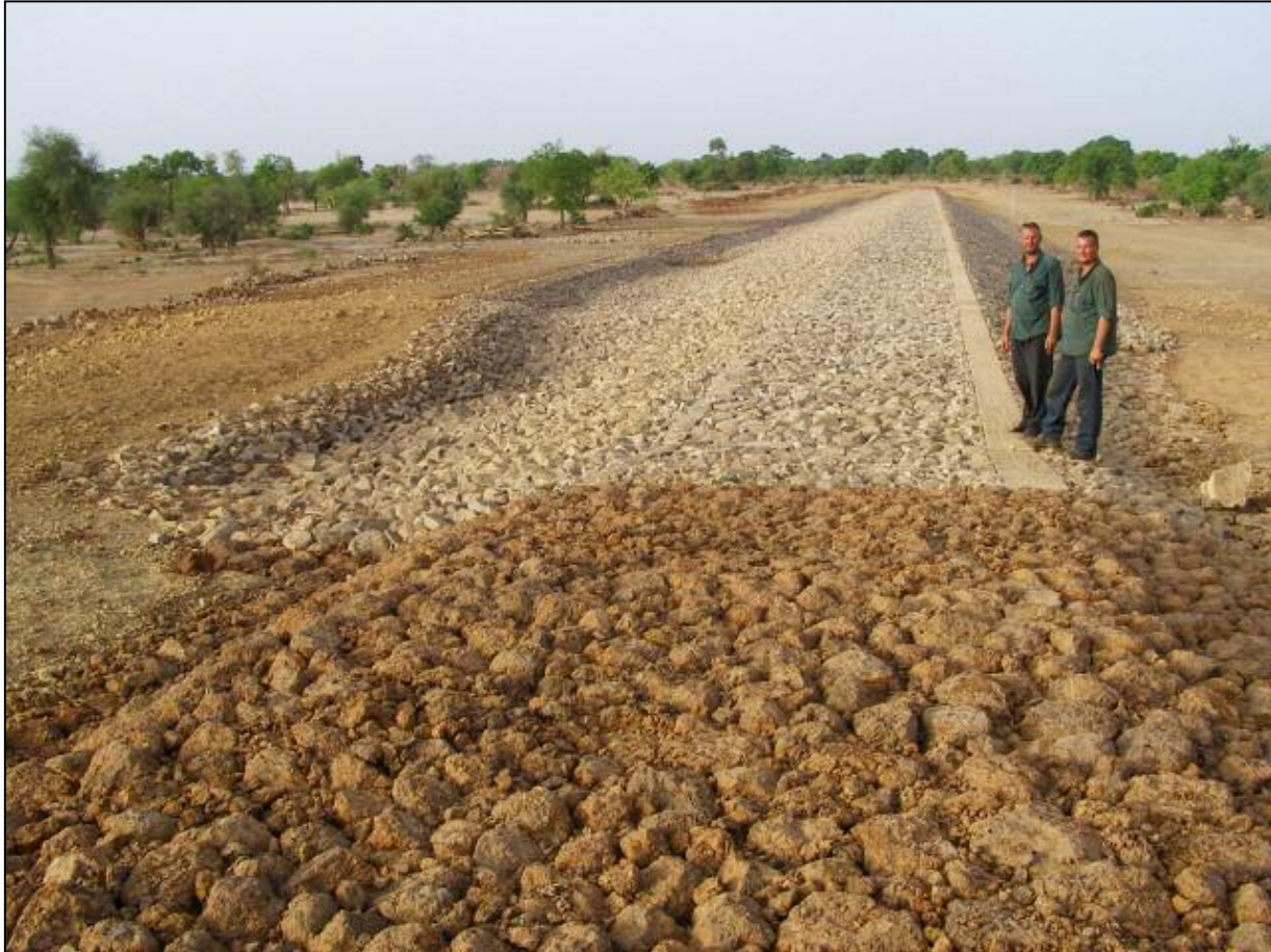
Figure 9: Combined Use of Granite and Laterite Rocks at the Tougoumatenga Spillway, Burkina Faso (2008)
