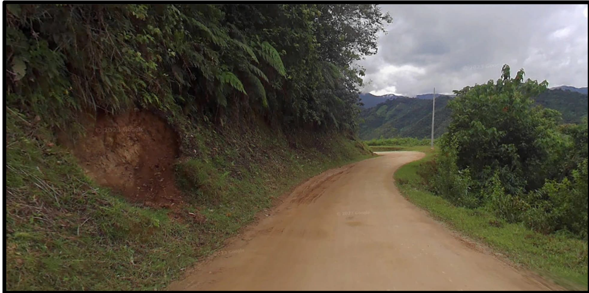
Figura 4.104. Talud inestable.
