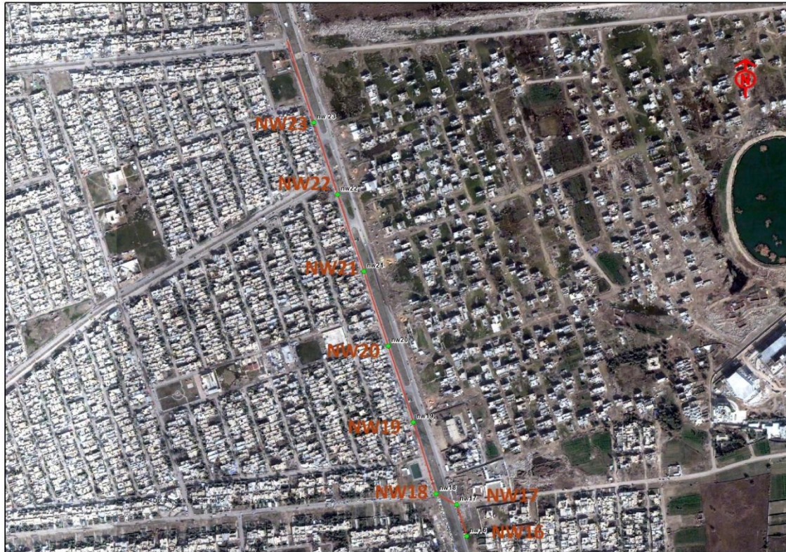
Figure 6: Collapsed main and manholes (NW16 – NW22)
