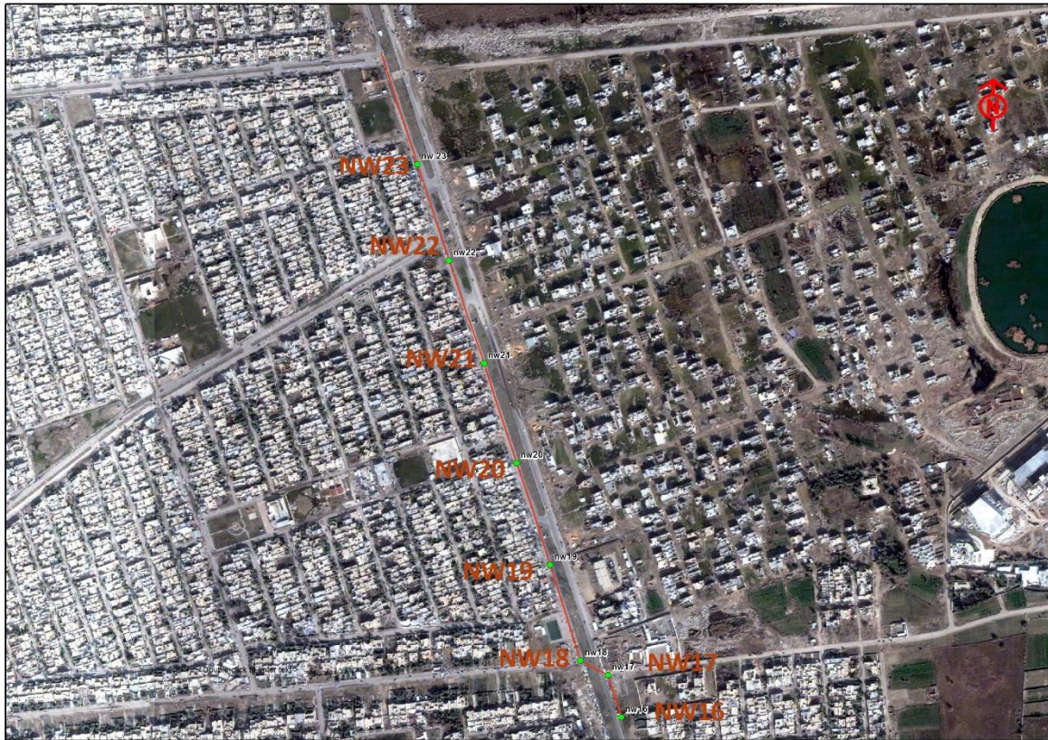
Figure 16: Collapsed main and manholes (NW16 – NW23)
