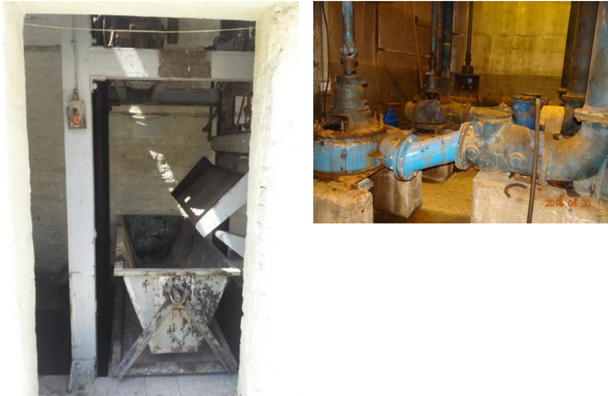
Figure 5: Current situation at Al-Habibiya SPS
