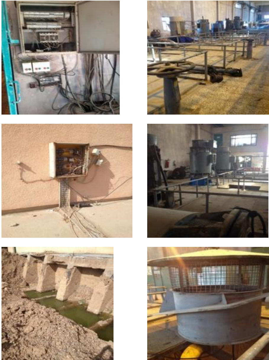
Figure 8: Current situation at Al-Doura 1 SPS
