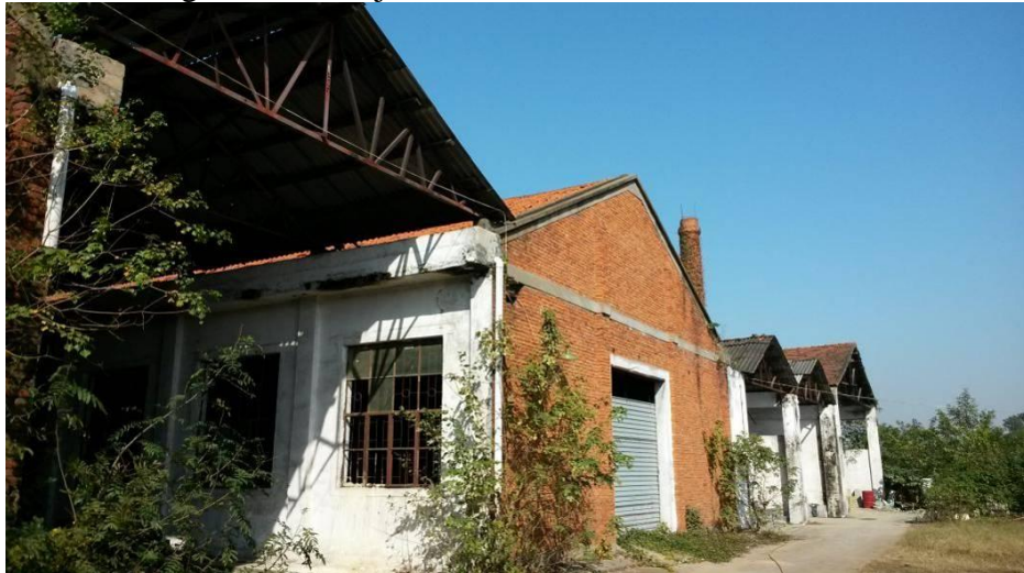
Figure 2-3: Several Warehouses of Chujin Iron Tower Co., Ltd. to be Demolished
