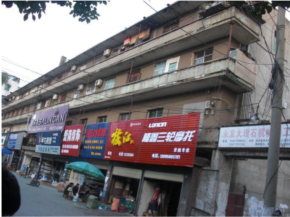
Figure 32-6: A Four-floor Building at No. 139, Handan Road to Be Demolished
