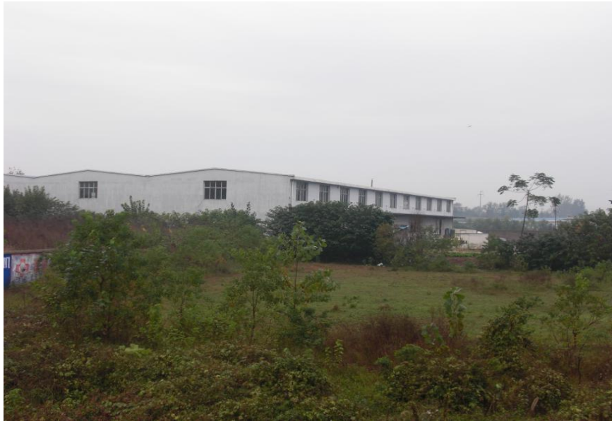
Figure 2-4: Warehouse of Hexie Logistics Company
