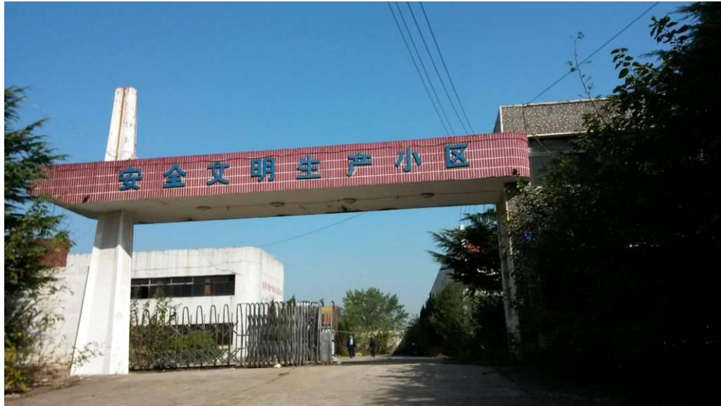
Figure 2-2: Chujin Iron Tower Co., Ltd. in Idle
