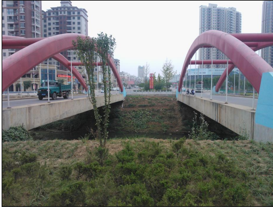
Fig. 2-2-3-4-3 Existing Condition of Jinqiu Avenue Where Crosses the Maohe River
