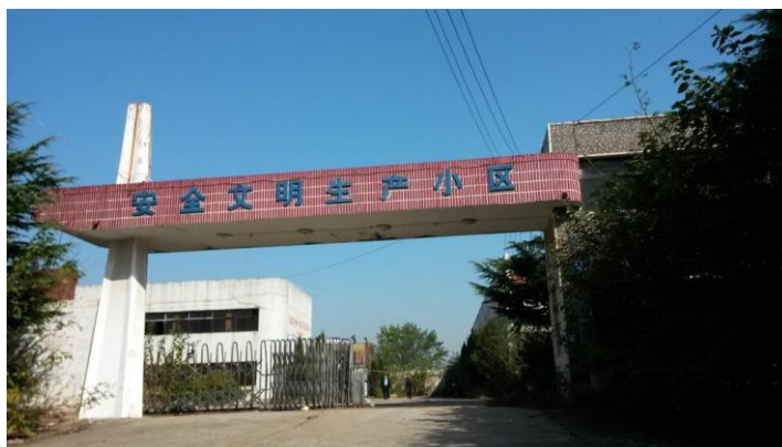
Fig. 3-3-5-1 Chujin Iron Tower Company in Bankrupt Idle Status
