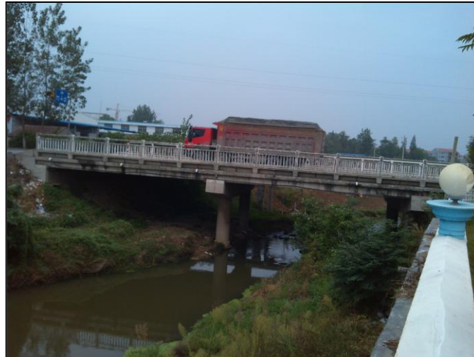
Figure 2-2-3-5-6 Current Situation of the Bridge Crossing Qili River on Yinxing Avenue
