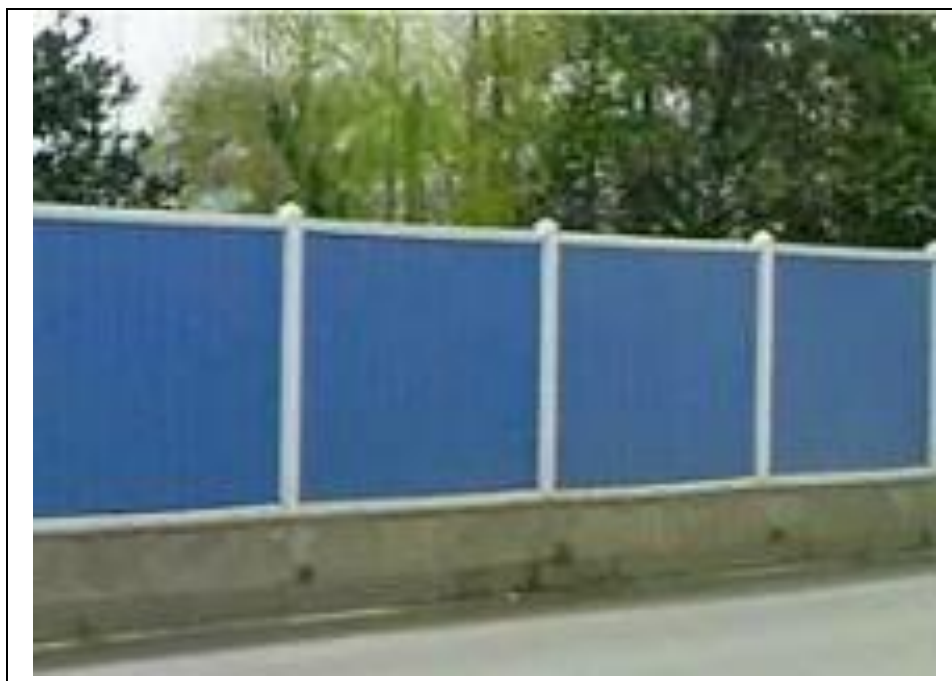
Fig. 5-1-2-3 Photo of Temporary Enclosure Boards for Similar Engineering
