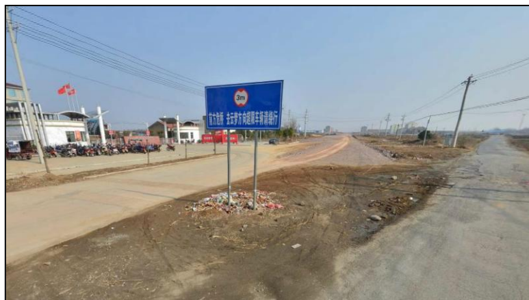
Fig. 2-2-3-2-6 Construction Site of Biyun Road (Everest Food Company ~ New G316)
