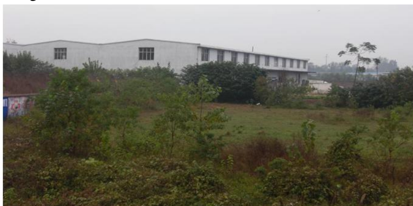
Fig. 3-3-5-2 Logistics Warehouse of Hexie Company
