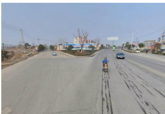
Intersection of Handan Road
