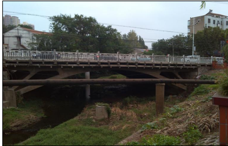
Fig. 2-2-3-3-3 Bridge Crossing Chashan River on Jiefang Avenue
