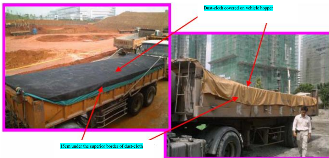
Fig.5.2-1 Sketch Map of Dust-cloth on Vehicle Hopper
