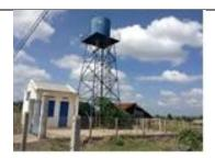
Headwork of a Community-based rural water supply using groundwater
