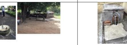
Shallow and deep groundwater wells. Proper ground sealing is important to prevent groundwater pollution caused by polluted surface water. Safety related to electrical wires would also be considered during operation
