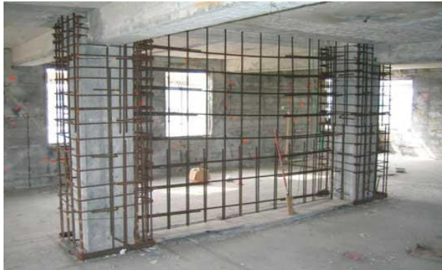
Figure 10-7: Retrofitting with RC shear-wall – before casting
