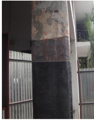
Figure 10-6: Column retrofitting with FRP
