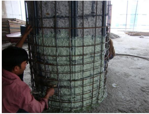
Figure 10-2: Column retrofitting with RC – before casting
