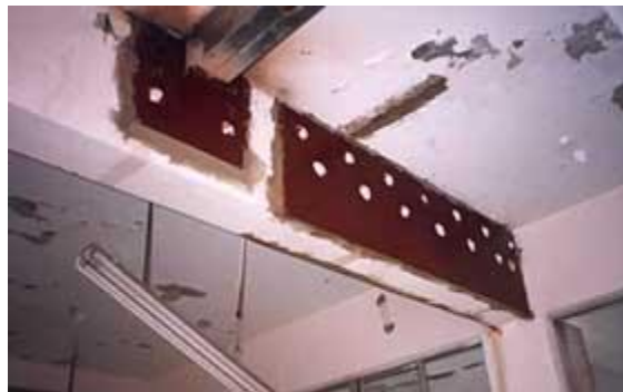
Figure 10-3: Beam retrofitting with steel plates
