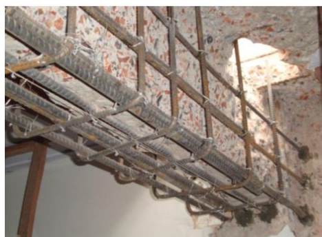
Figure 10-1: Beam retrofitting with RC – before casting
