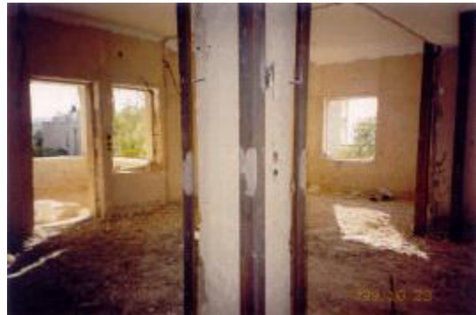
Figure 10-4: Column retrofitting with steel angles
