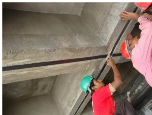
Figure 10-5: Beam retrofitting with FRP
