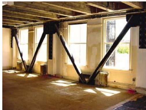
Figure 10-8: Retrofitting with steel bracing
