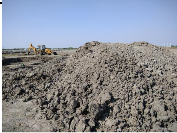
Photo 7: Excavation work at Balledupalle site
