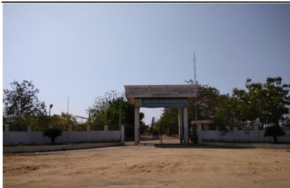
Figure 2.5 Substation at Veltoor
