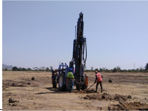
Photo 8: Piling work at Addakal site
