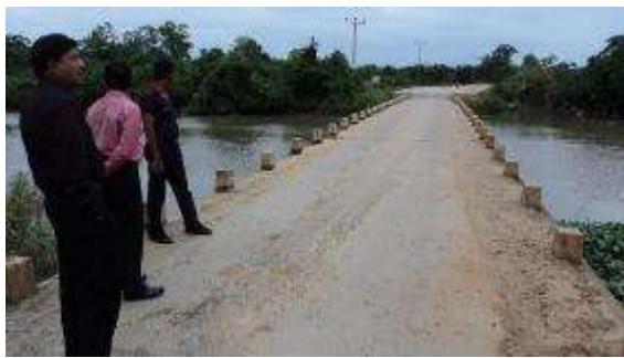
Existing bridge at Sungawila
