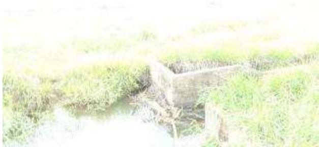
Flood damage to canal structures Bottleneck for efficient water movement
