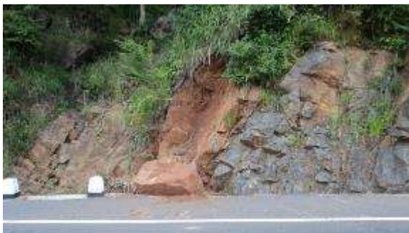
Falling rock boulders at 60/3
