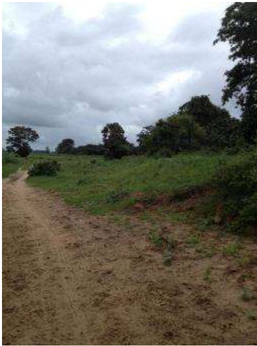
Flood bund that requires improvements
