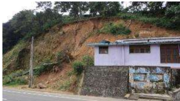
House threatened by landslide at 46/2
