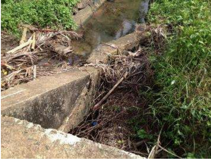
Collapsed structures of Allai scheme
