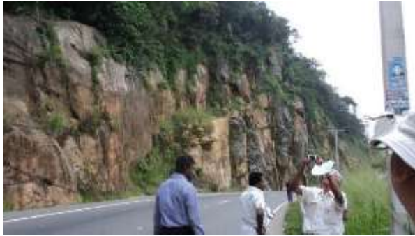
Hanging rock boulders at 55/4
