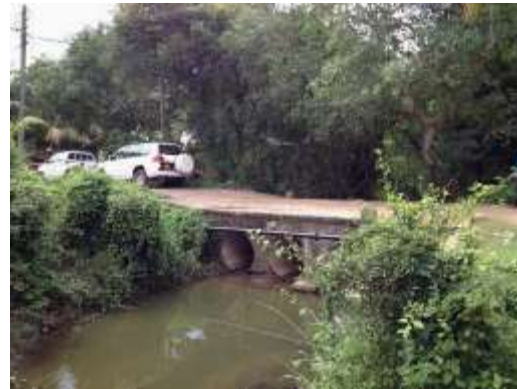
Low capacity culvert
