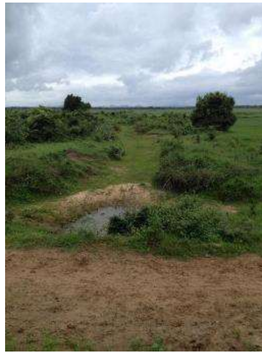
Silted and collapsed canal
