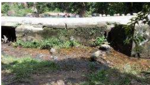
Damages to the causeway
