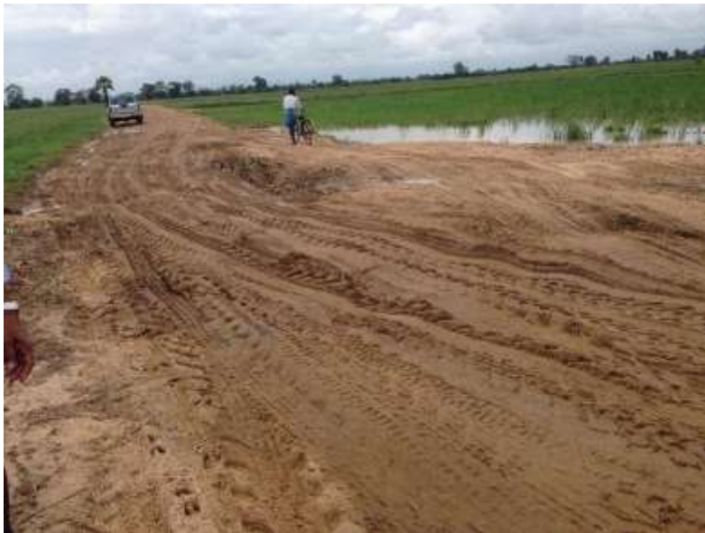
The ID gravel road that gets flooded and eroded
