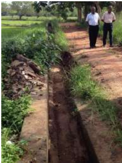
Damaged field canals
