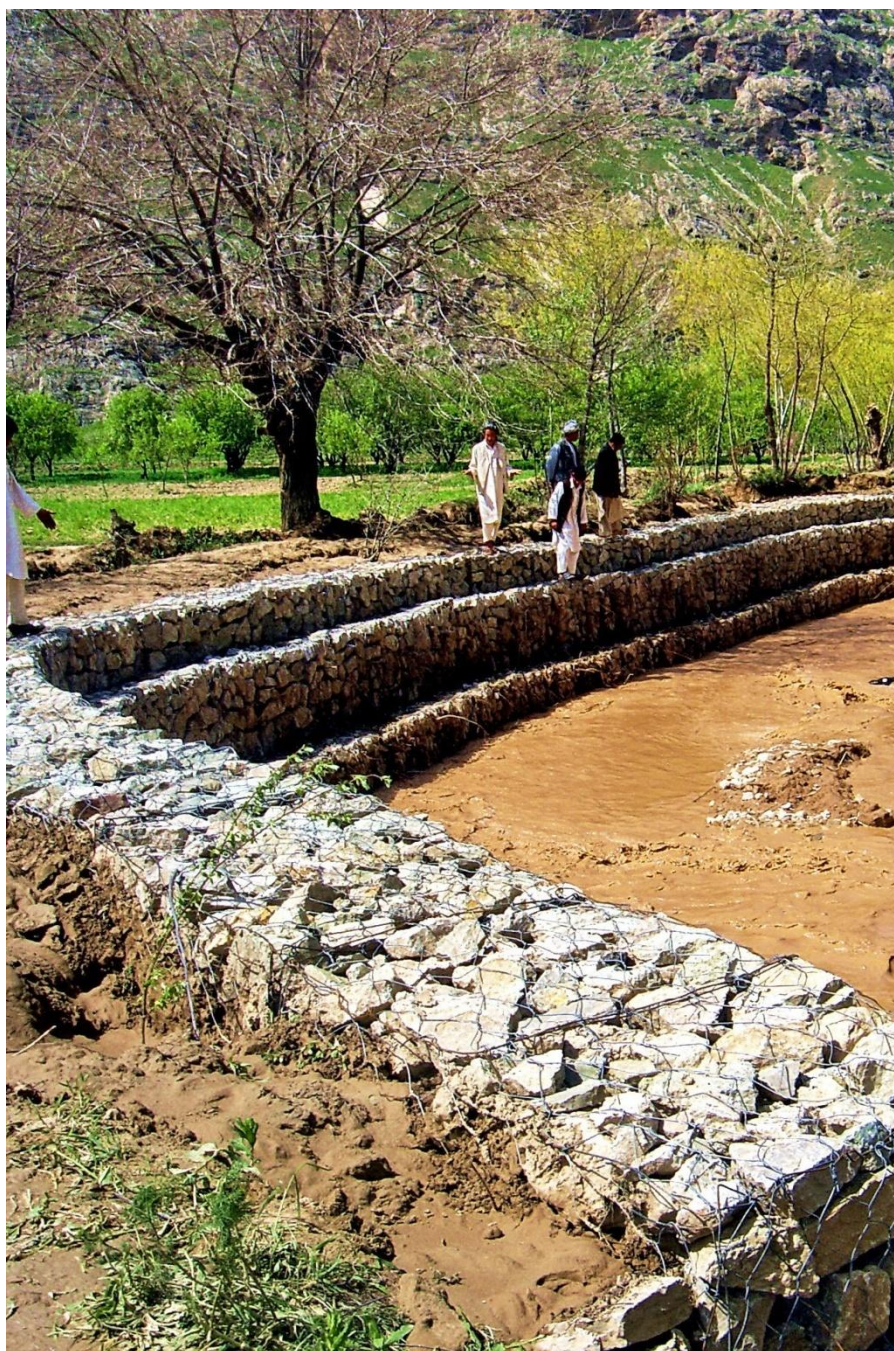
river bank protection to control erosion and contributes to safe farming
