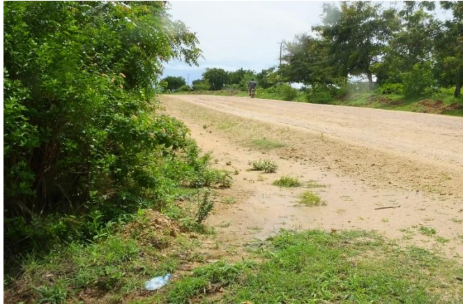
Figure 4.4: Tanga-Pangani trunk road and Electric transmission near the site
