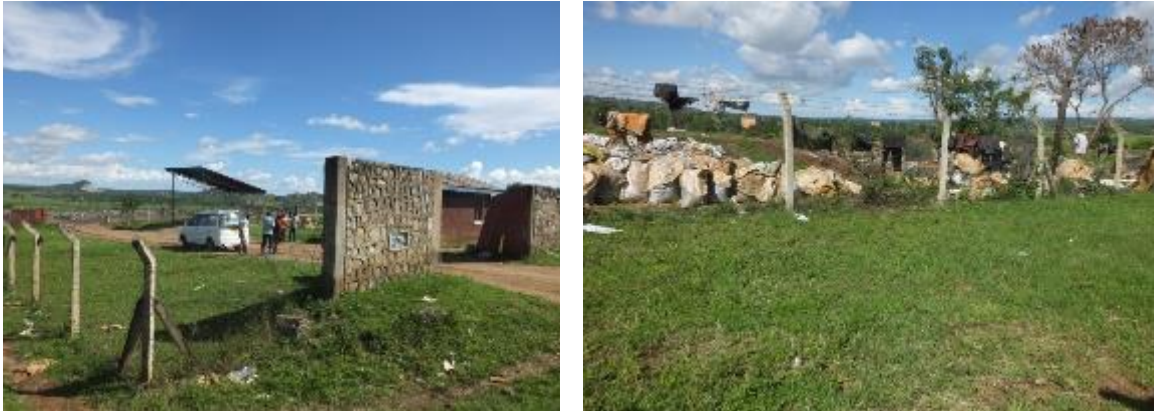
Figure 4.4: Existing structures at the project site
