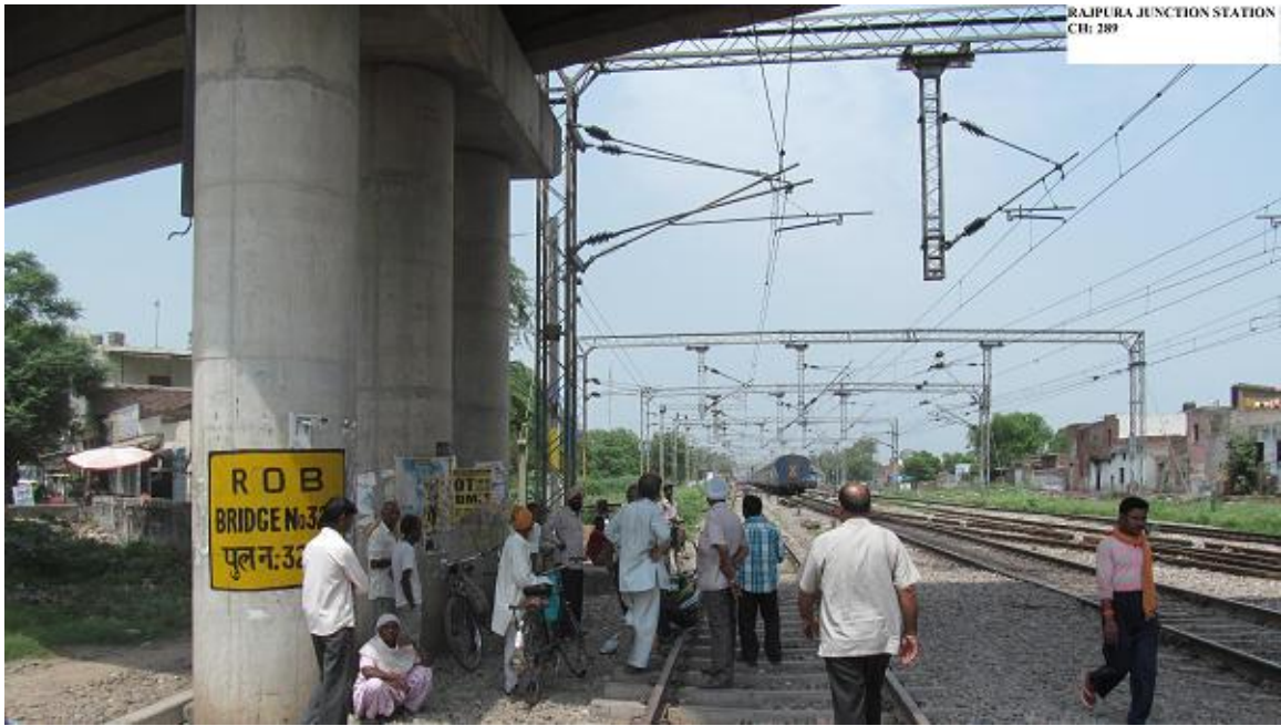
Figure 2.16 : View of Rajpura Junction Station (Above)
