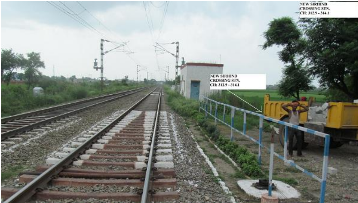
Figure 2.14 : Site for New Sirhind Crossing Station
