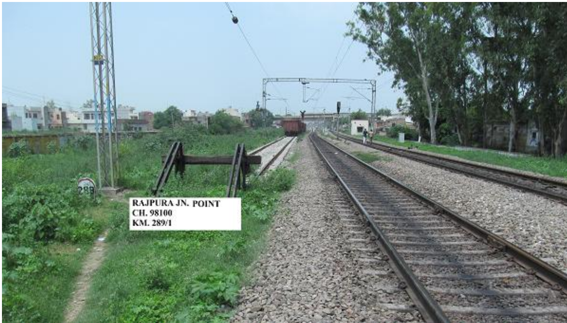
Figure 2.10: Location of Rajpura Junction Point
