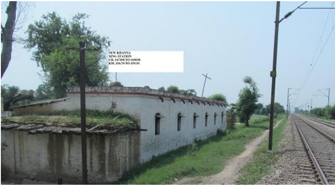
Figure 2.8: Site for New Khanna Crossing Station
