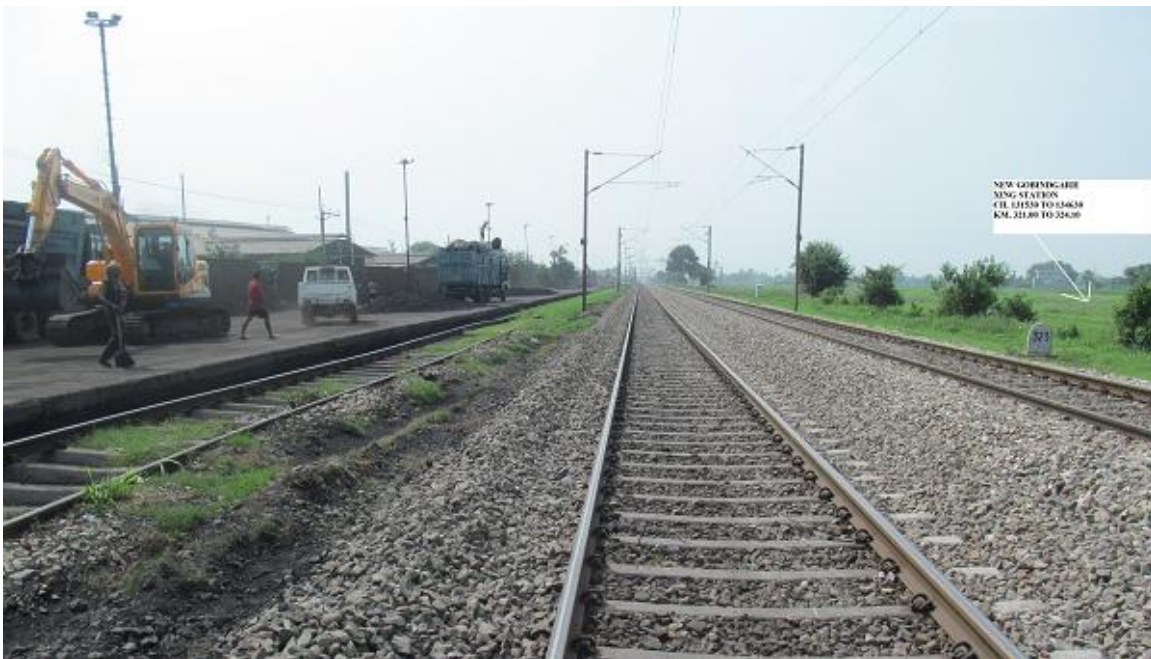
Figure 2.9 : Site for New Govindgarh Crossing Station
