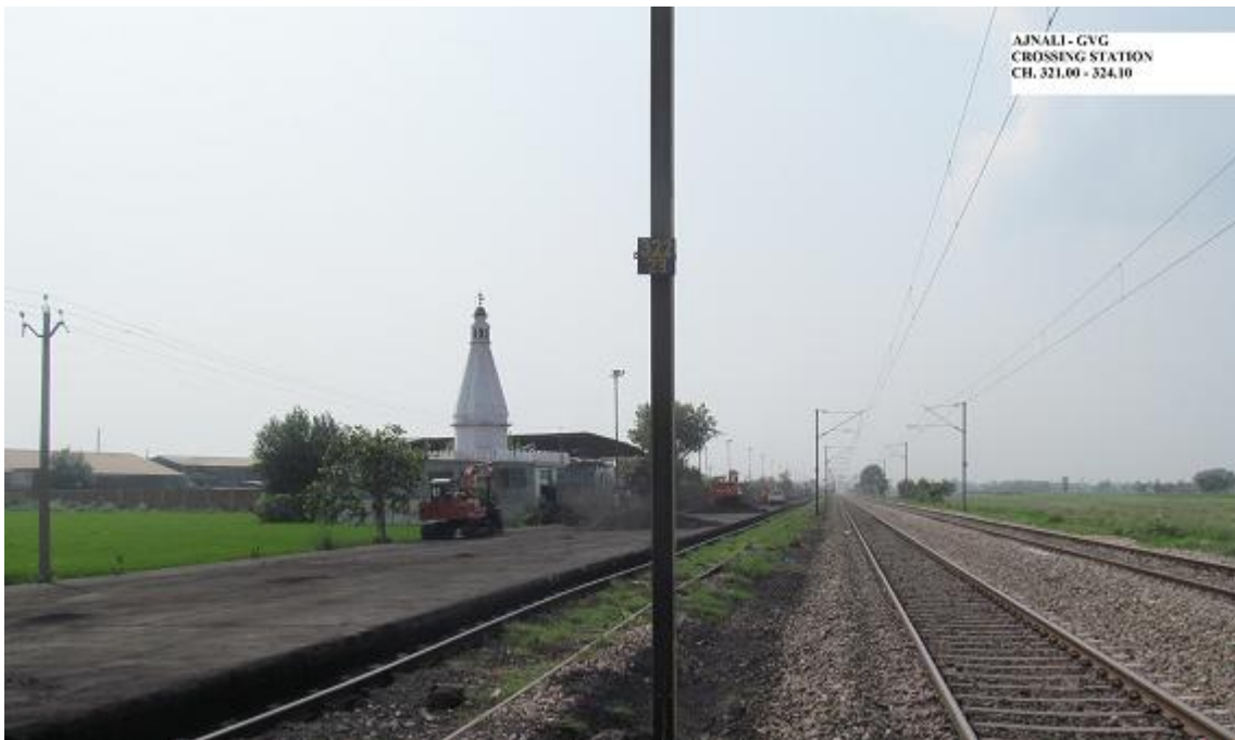
Figure 2.15 : Site for New Govindgarh Crossing Station
