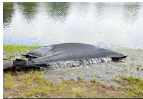
Plate 3.2 Silt bag under inspection
