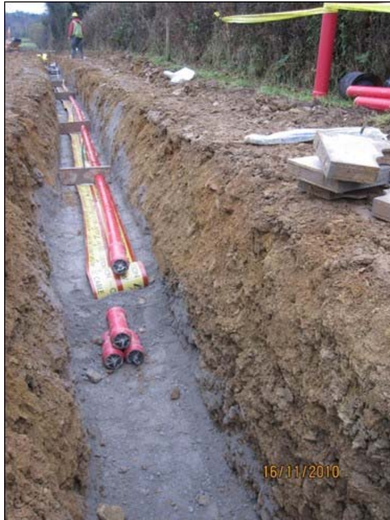
Plate 2.1 Cable Trench View
