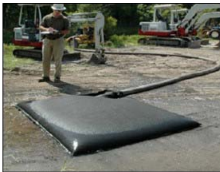
Plate 3.1 Silt Bag with water being pumped through
