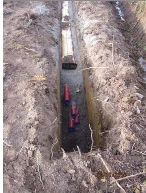
Plate 2.2 Cable Trench View
