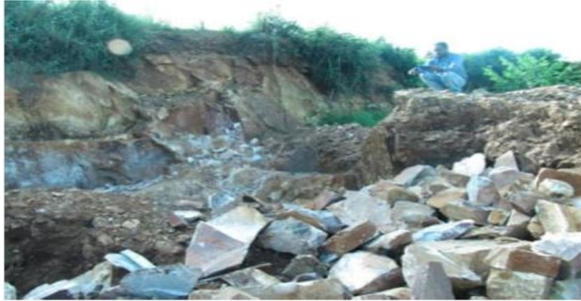
Plate 3-4: Munege rock quarry, Km 20+100, RHS, Offset 300m (Whitish grey quartzite and granitic)
