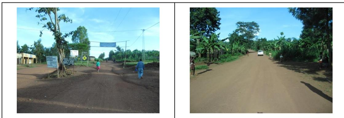
Figure 5-4: Pronounced rutting, loss of camber and lack of side drainage system
