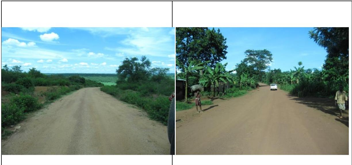
Figure 3-3: Fair condition of carriageway but side drains and bridge insufficiently maintained
