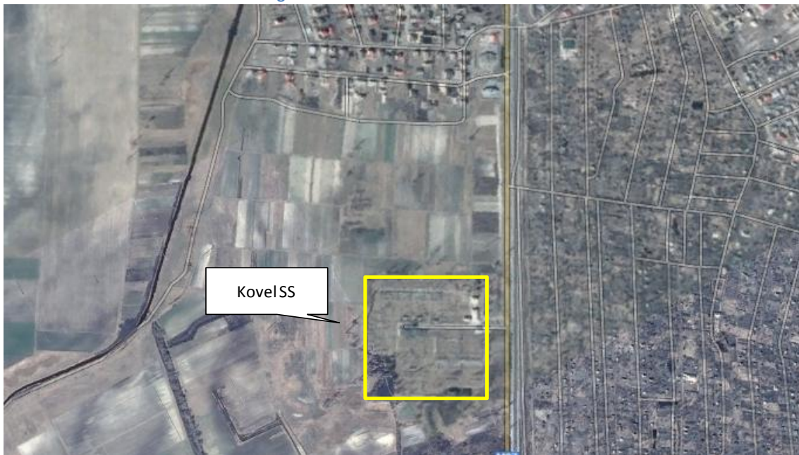
Figure 36 Location of Kovel Substation
