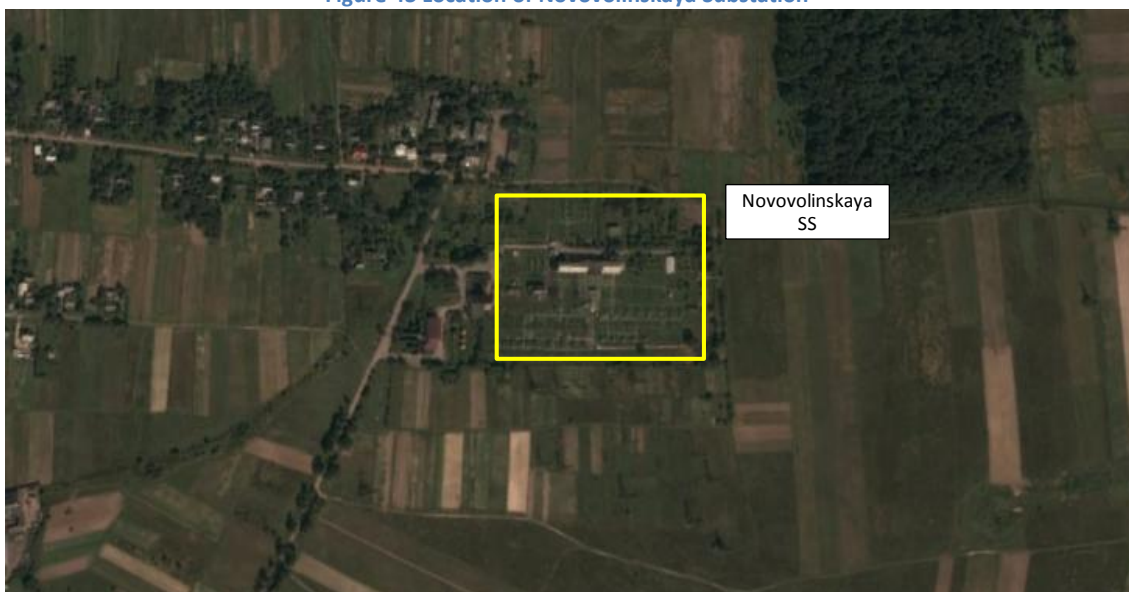
Figure 43 Location of Novovolinskaya Substation
