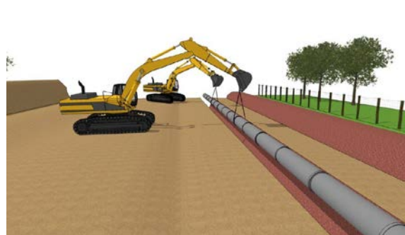
Figure 2.4 Welded Pipe String Installation
