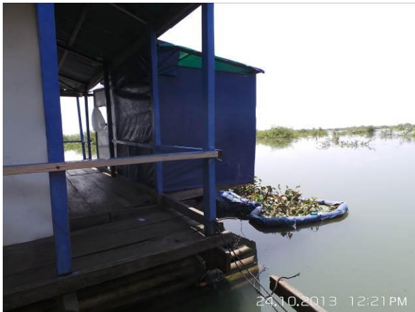
Toilet introduced by Wetlands Work in Akul Village
