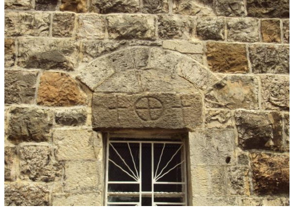
Engraved lintel over one of the windows
