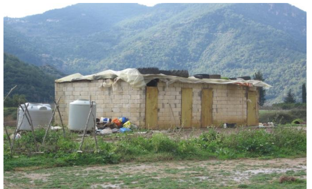
Housing for seasonal farm workers
