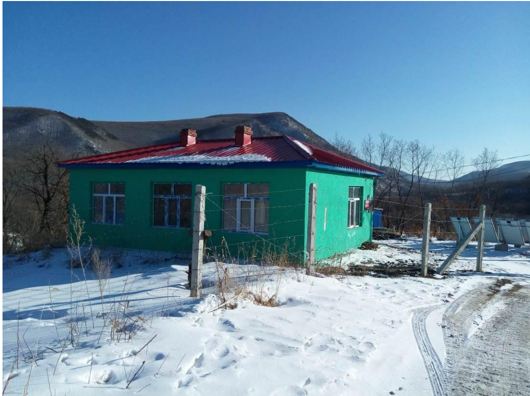
Figure 2-1: Example of Newly-build Protection Station
