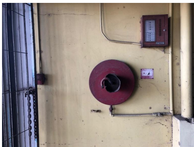
Figure 7.4: Missing Fire Hose
