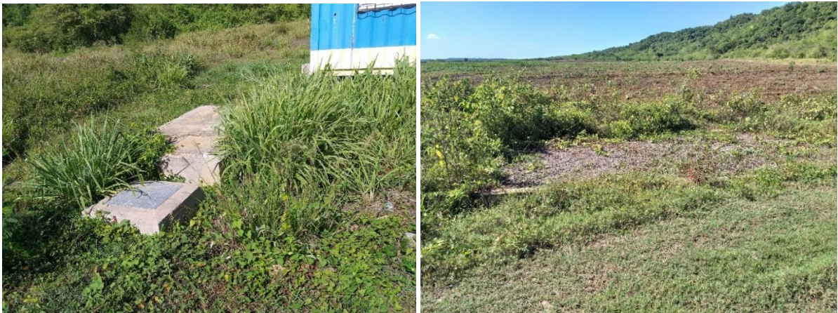
Figure 5.6: Septic tank at SPAP (left); Reed Bed at SPAP (right)
