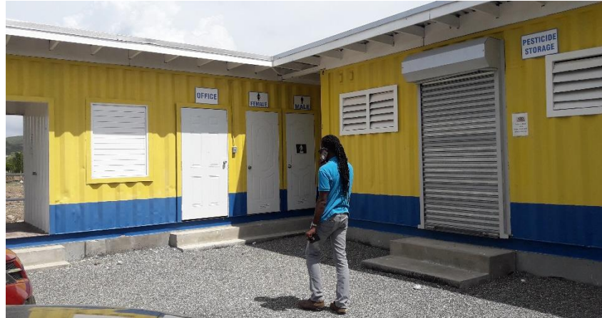
Figure 4.4 Yallahs Agro Park Packaging Facility
