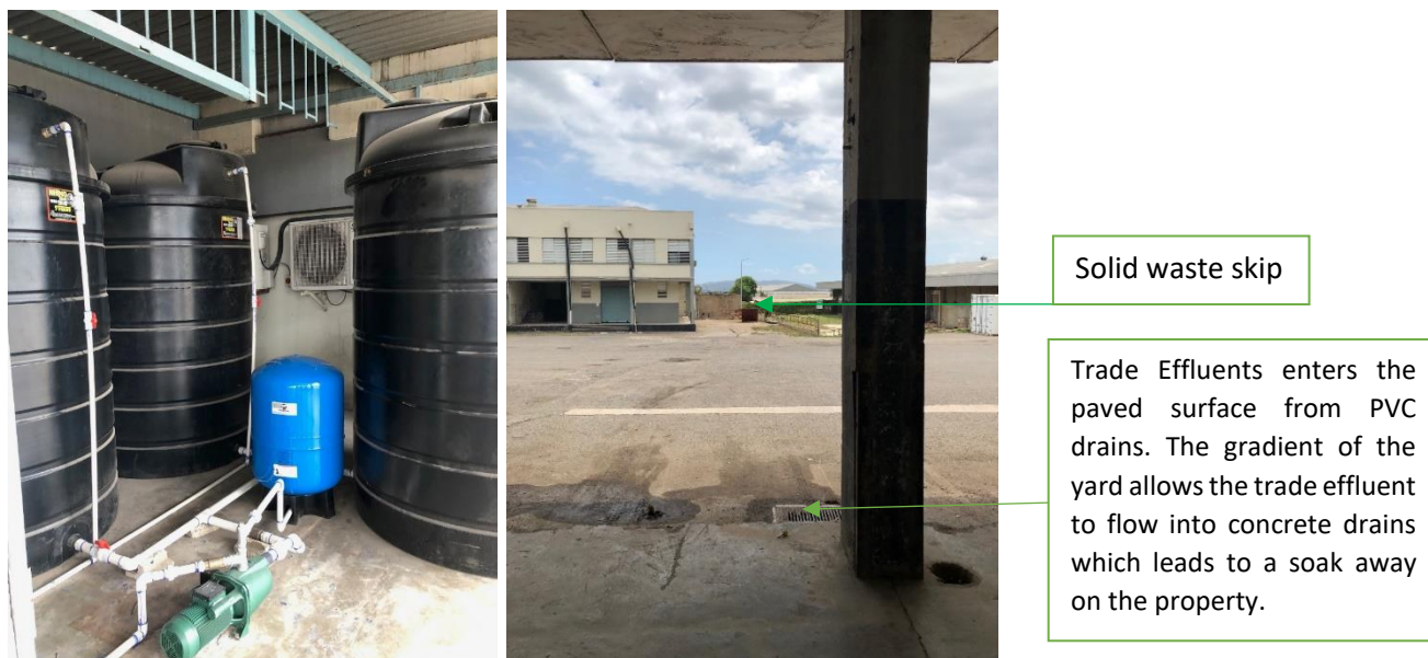
Figure 7.3: Potable Water Storage Tanks and Distributing System (left); Skip for solid waste (right); Drain for Trade Effluent (right)
