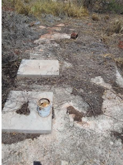
Figure 6.4: Septic Tank at NFDH Packing Facility
