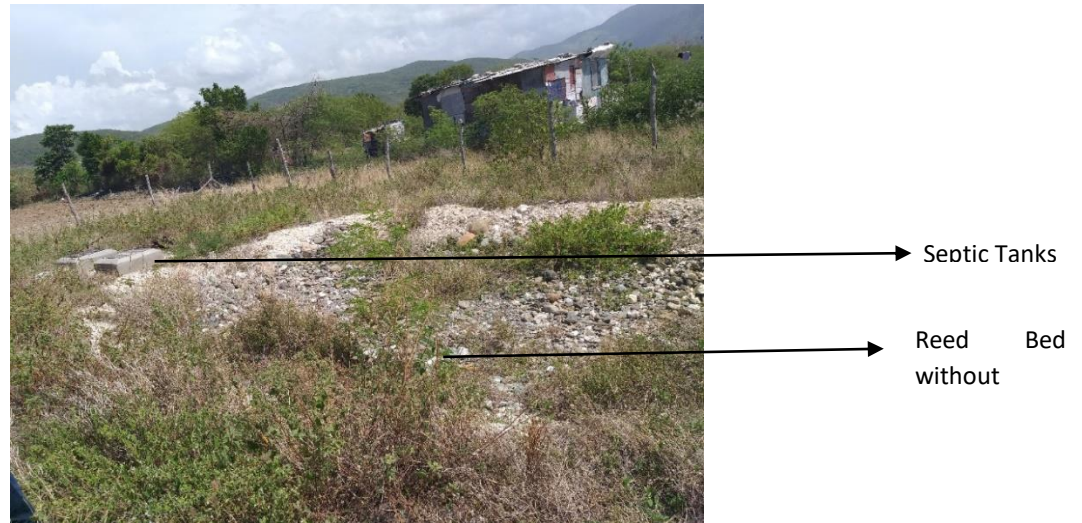
Figure 4.6: WWT System at Yallah Agro Park showing Septic tanks and Reed Bed
