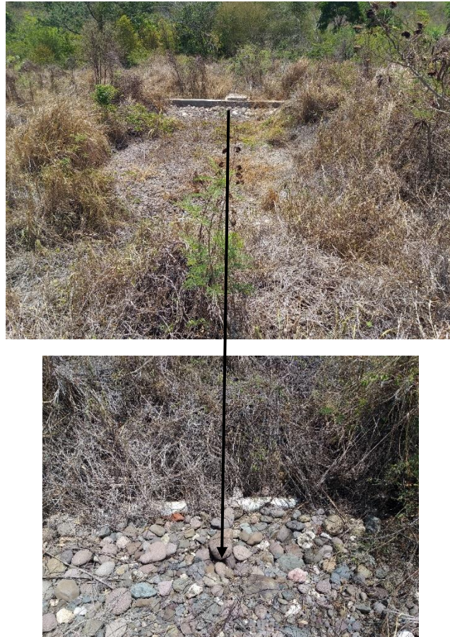
Figure 6.5: Reed Bed (without reeds) at NFDH Packing Facility
