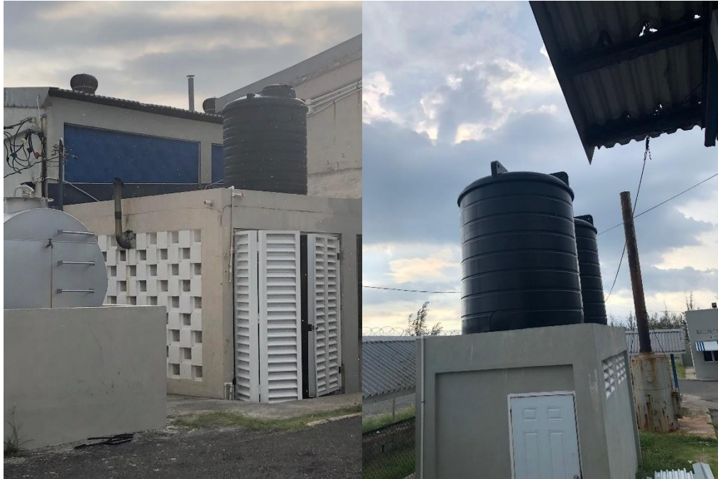
Figure 7-13: Potable Water Storage Tanks
