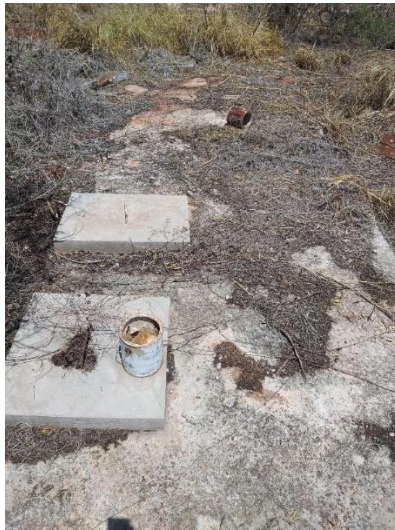
Figure 6.4: Septic Tank at NFDH Packaging Facility
