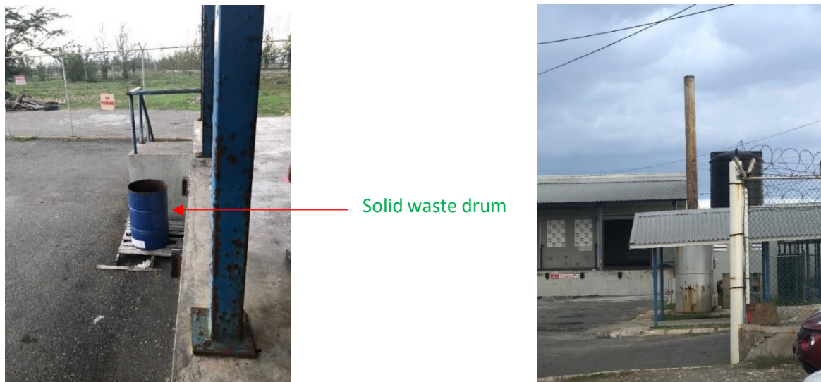
Figure 7-15: Drum for solid waste (left); Incinerator (right)
