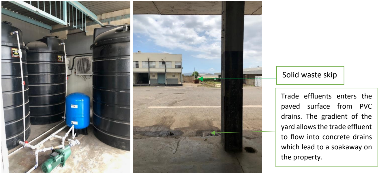
Figure 7.3: Potable Water Storage Tanks and Distributing System (left); Skip for Solid Waste (right); Drain for Trade Effluent (right)
