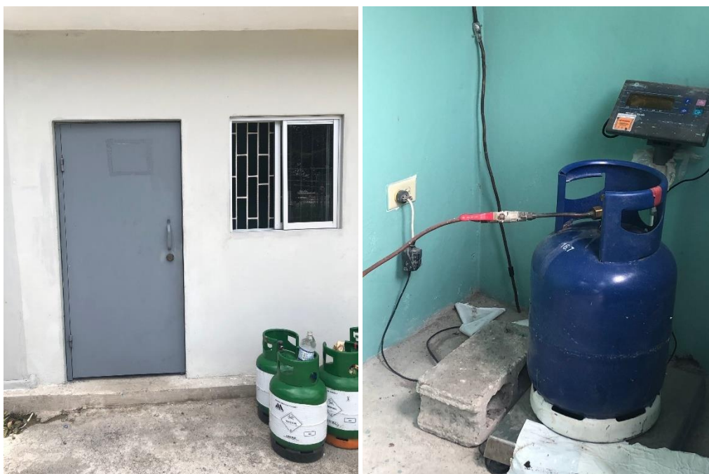
Figure 7-35: Gas Delivery Room (left) Unsecured gas cylinder (right)
