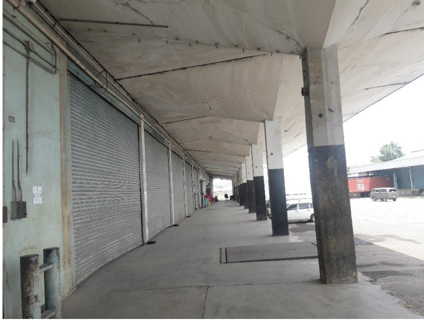
Figure 7.2: Deteriorated Building on the AMC Complex
