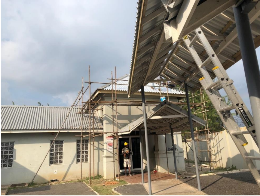
Figure 7-9: Repair of Roof
