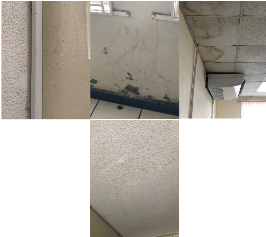
Figure 7-10: Signs of Moisture Intrusion inside Building
