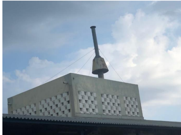
Figure 7-21: Exhaust Stack for Fumigation Rooms
