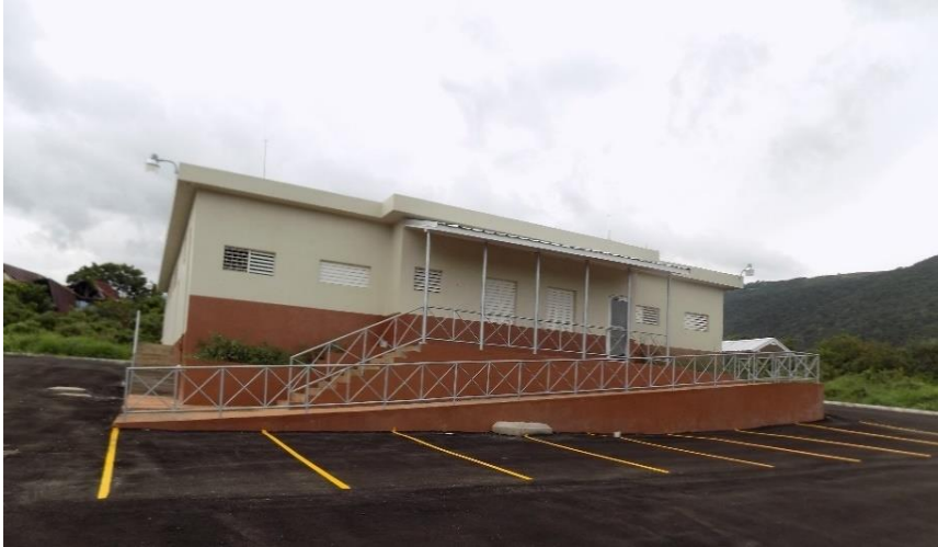
Figure 6.3 Complete Packaging House in the NFDH Agro Park
