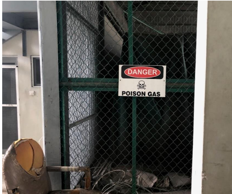
Figure 7-33: Signs by Fumigation Station
