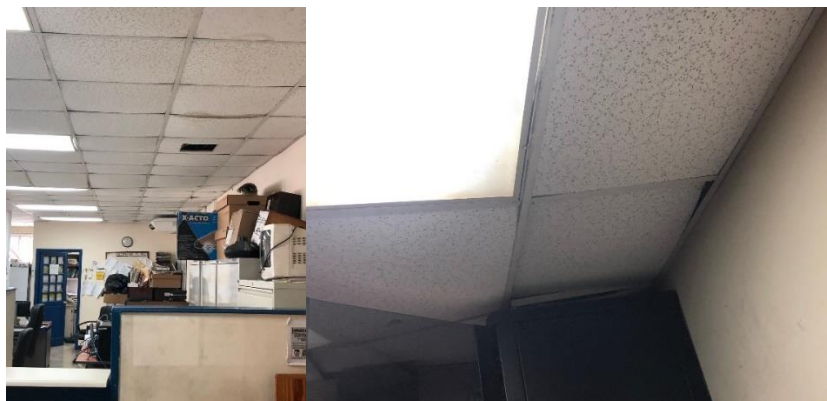
Figure 7-12: Unseated and Missing Ceiling Tiles
