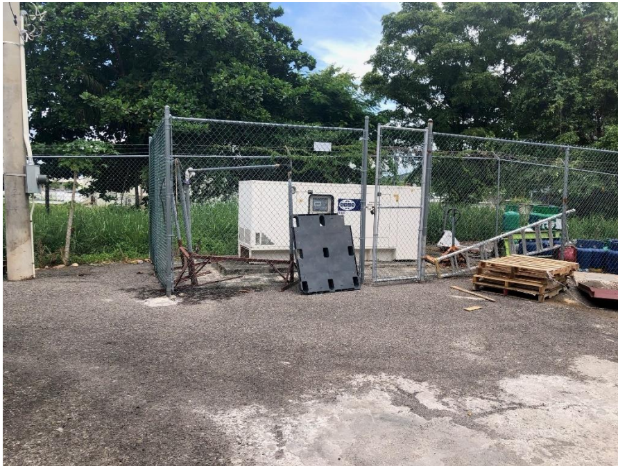
Figure 7-27: Backup Generator for Fumigation Facility
