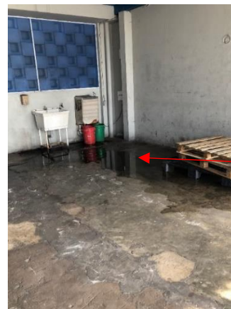
Figure 7-17: Ponding Water on AEC
