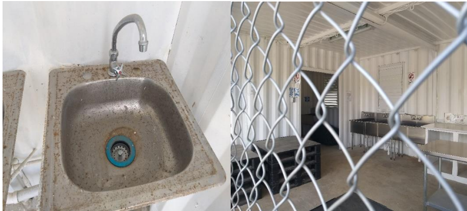
Figure 4.5 Rusting Metal Works at Yallahs Agro Park Packaging Facility
