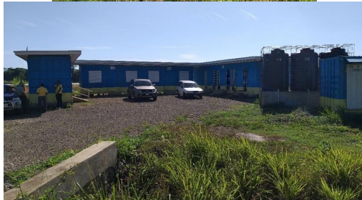
Figure 5.4 Spring Plain Produce Handling Facility
