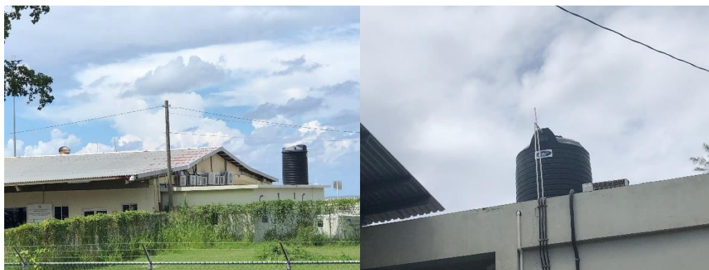
Figure 7-28: Potable Water Storage Tanks
