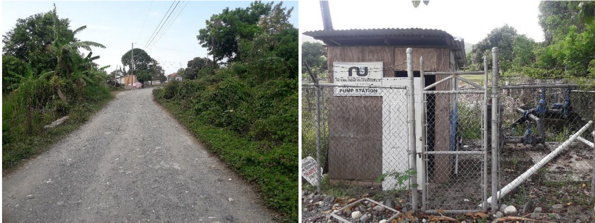
Figure 4.3: Road and Irrigation Infrastructure constructed in the Yallahs Agro Park
