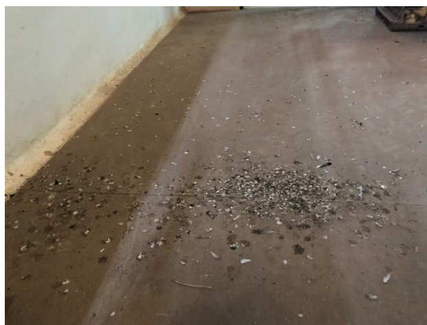
Figure 7.6: Pigeon Droppings inside the Packing House
