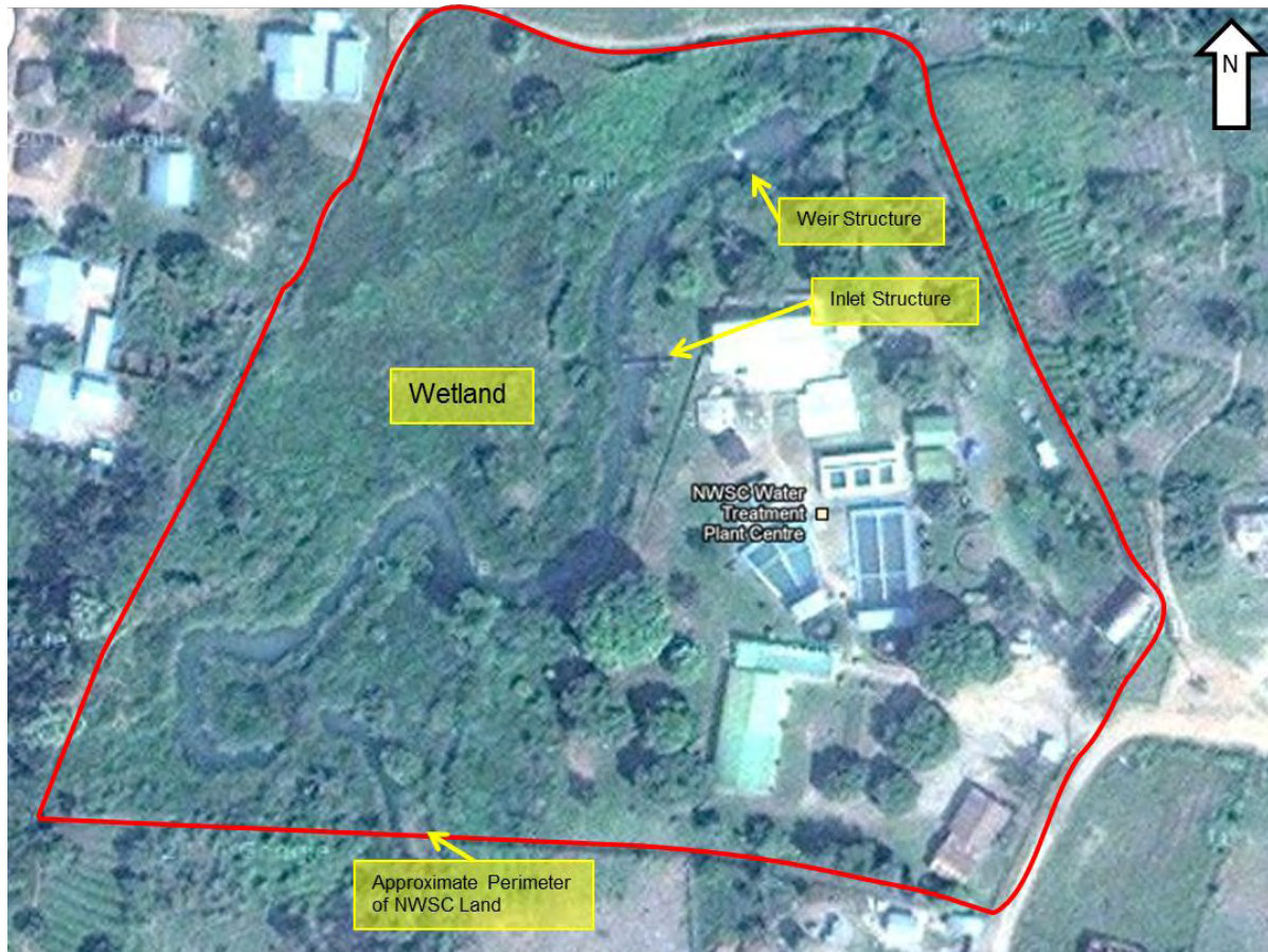
Figure 1: Arua WTW, River Enyau and Wetland
