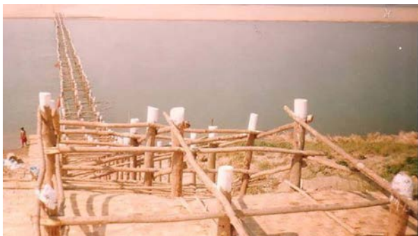
Figure 4 Examples of local timber pile groynes
