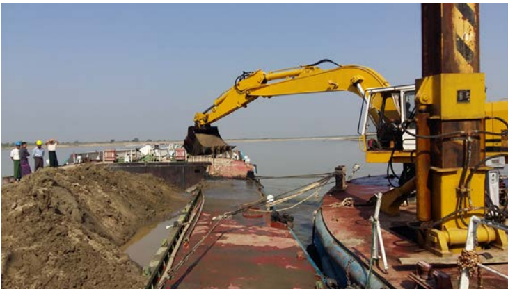
Figure 6 DWIR Backhoe dredge
