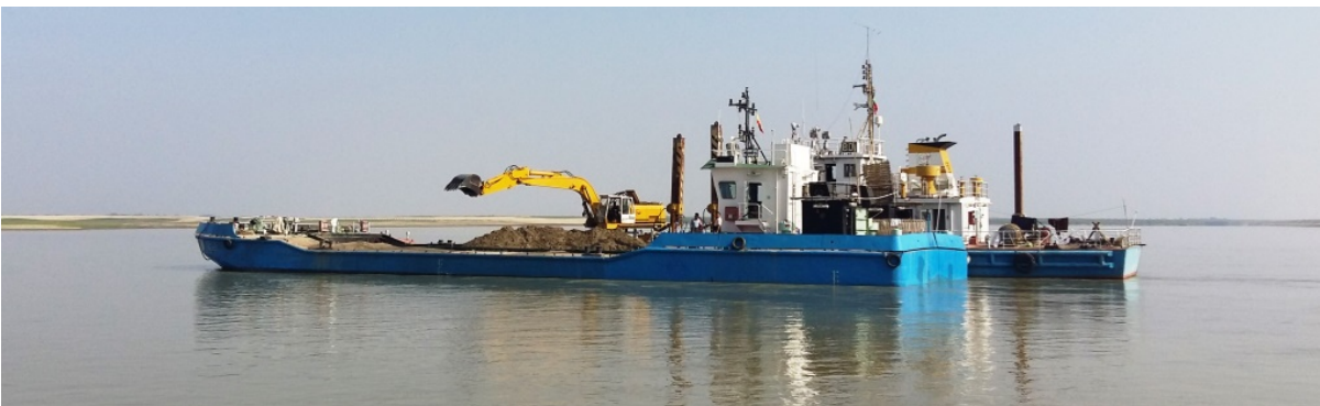
Figure 7 DWIR Split barge
