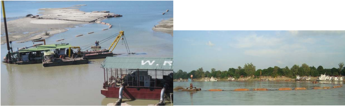
Figure 5 Cutter Suction Dredger with floating pipes
