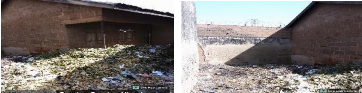
Plate A.2: Front view of the student’s toilet at GDSS Pantami
