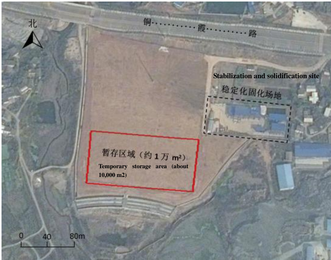
Figure6.6-5 Location map for temporary storage site
