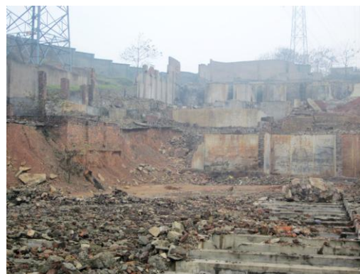
d. Part of Tongda Smelting Plant
