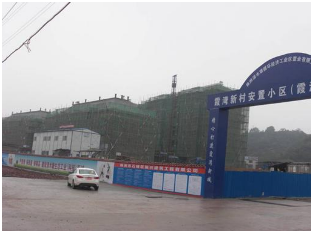
Figure12.1-5 1 st Resettlement Houses in New Xiawan Village are Roof Sealed
