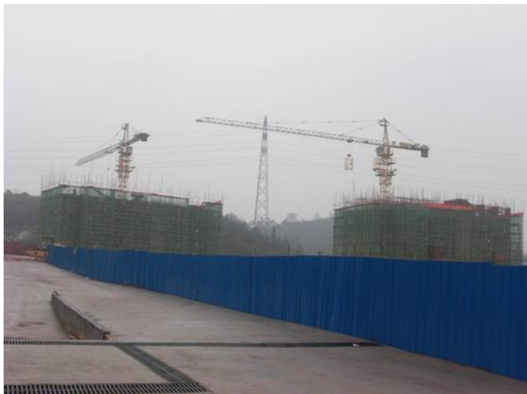
Figure 12.1-6 2 nd Resettlement Houses in New Xiawan Village are under Construction
