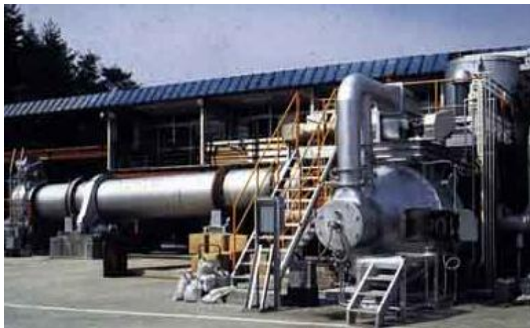
Figure 8.3-6 Incineration in rotary kiln
