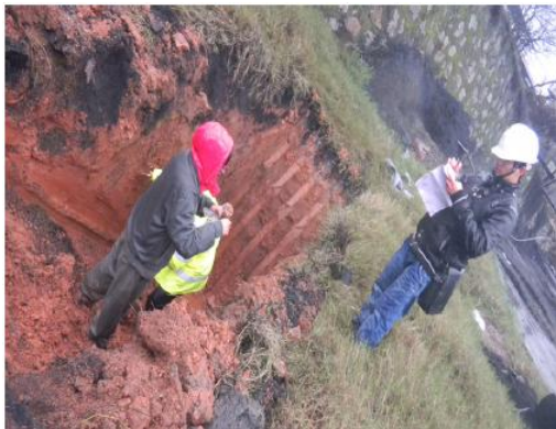
g. Excavated section of Dongtai Industry Co., Ltd.
