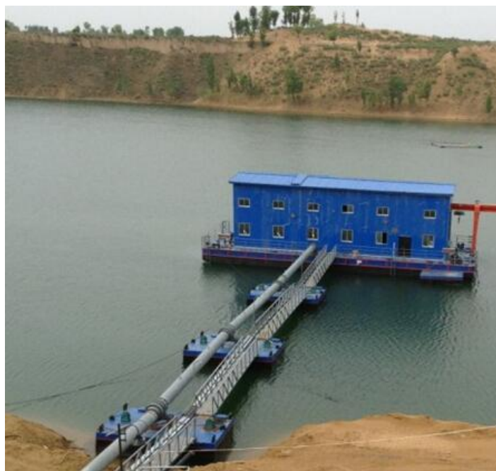
Figure6.10-2 Diagram for pontoon pump station
