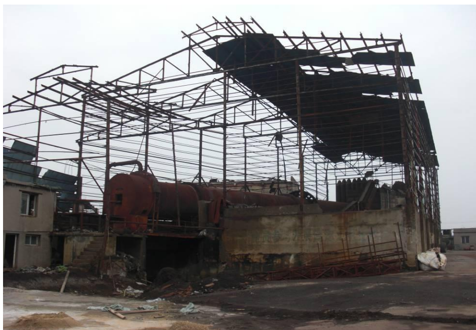
Picture 6-1 buildings to be demolished in the Yongfa refinery
