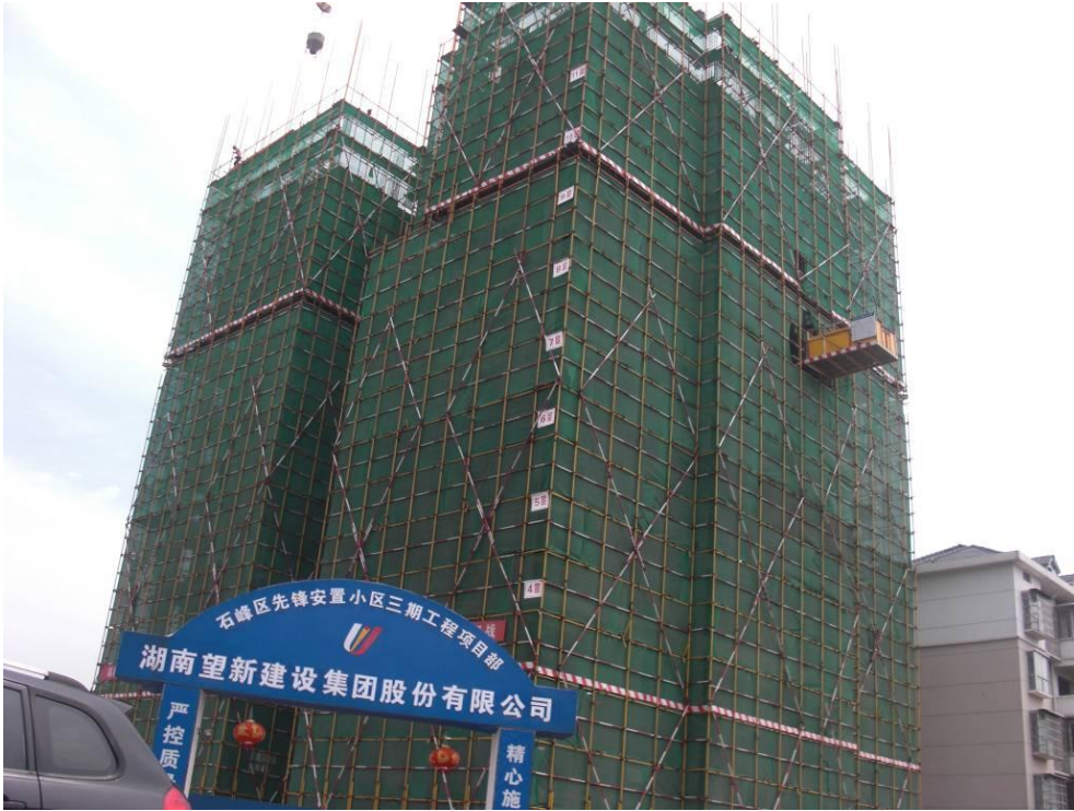
Picture 5 Xianfeng Resettlement Community to be delivered for use in April, 2016
