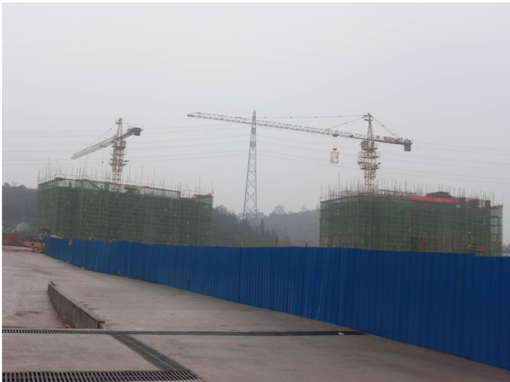
Picture 6-2 Construction of Second-phase Resettlement Housing in Xiawan Residential Quarter is Underway
