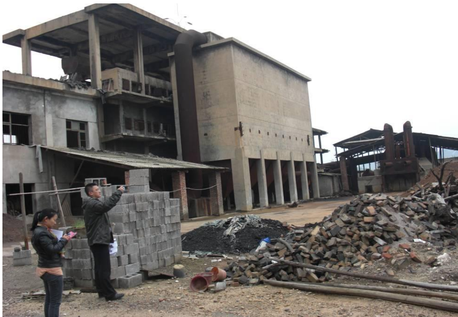
Picture 6-2 Buildings to be Demolished in the Area of Kangli Smelting Plant
