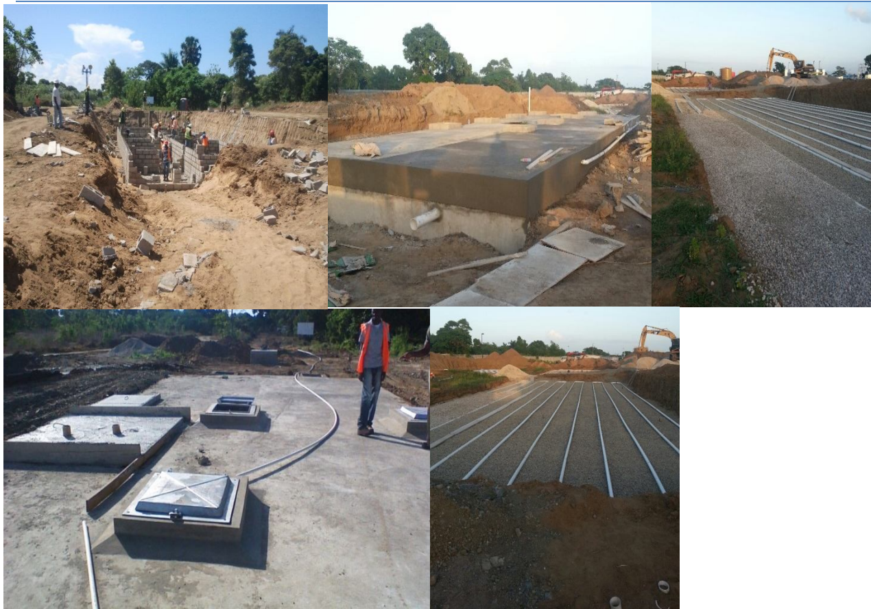
Figure 15: Views of the Septic Tank and Drainage Field at WWTP#2 during construction (IDB)
