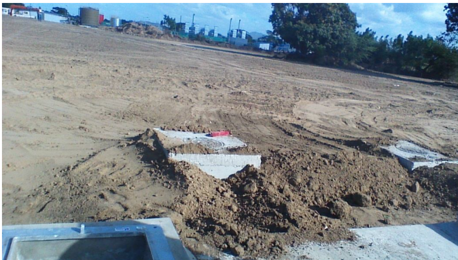
Figure 14: Showing completed drainage gallery viewed from the septic tank at WWTP#2
