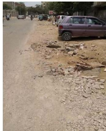
Figure 5.5: Picture of ill maintained newly buried sewerage line at Strachan road with open manhole
