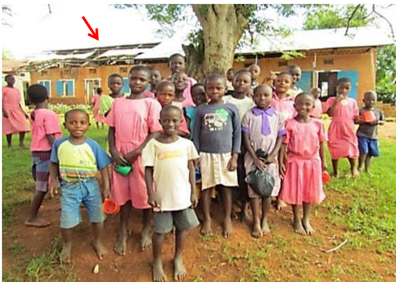
Plate 4: Rehabilitation of classroom blocks such as this rural primary school building with part of its roof blown off (left background) would ensure safety of pupils and teachers
