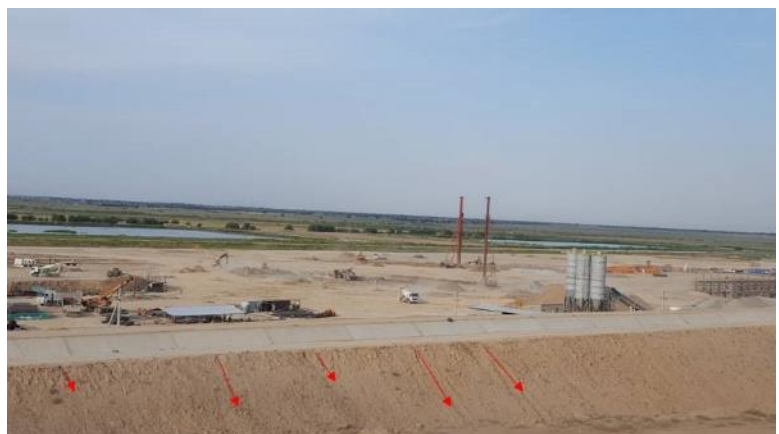
Figure 9.3.3: Rill-washing erosion of fill material at the Project Area (Ramboll Photos on July 08 th , 2019)
