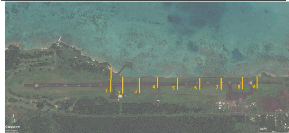
Figure 2: Location of nine current culvert drains under the runway (Source: Google Earth Pro, dated April 2015)
