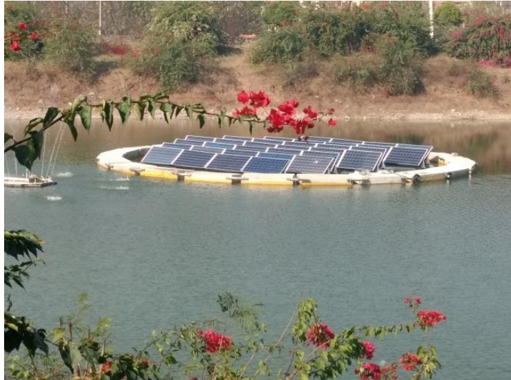
Figure 1-3: Floating Solar 10 Kw (Chandigarh)
