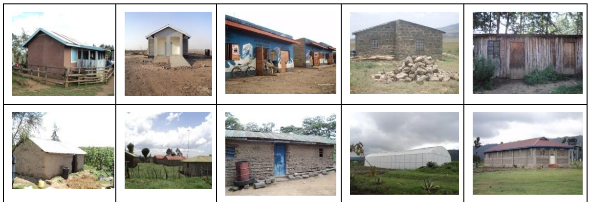
Fig. 7.1 - Some of the Affected Structures
