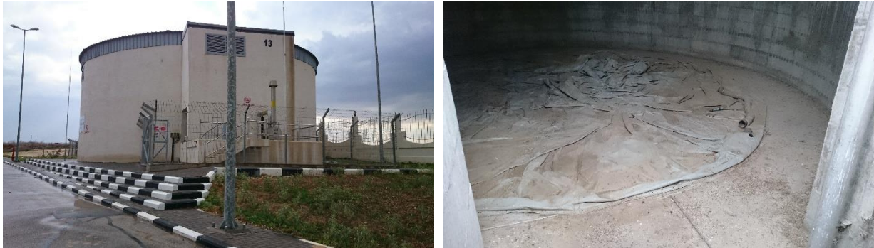
Figure 2-2: The biogas balloon site at NG WWTP
