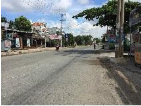
Access road of Dong An residence area
