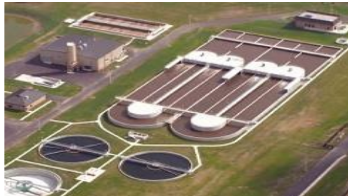
Figure 6-2 Oxidation ditches technique
