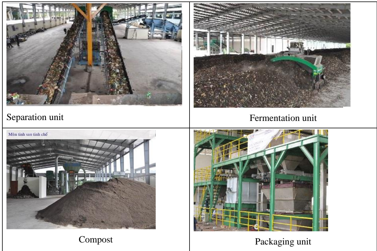
Figure 4-10 Photos of Composting Plant at Binh Duong SW Treatment Complex
