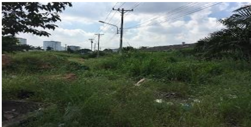
Picture 5. 1. Electric line over the region of pump station G1-1
