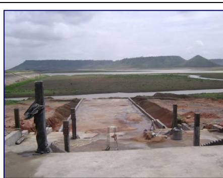
View of Mohini Weir
