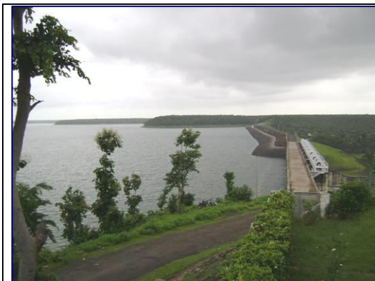
View of Kolar Dam
