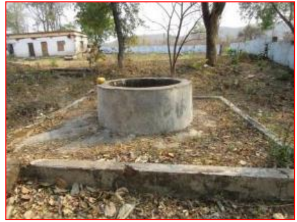
Project Affected Open Well
