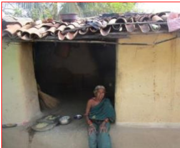
Residential House going to be dismantled
