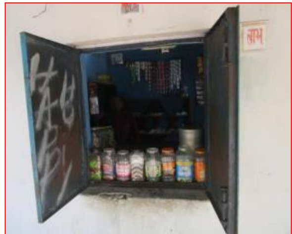
Residential cum. Commercial House going to be dismantled
