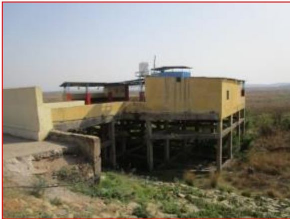
Project Affected Cremation Structure at Gandhinagar
