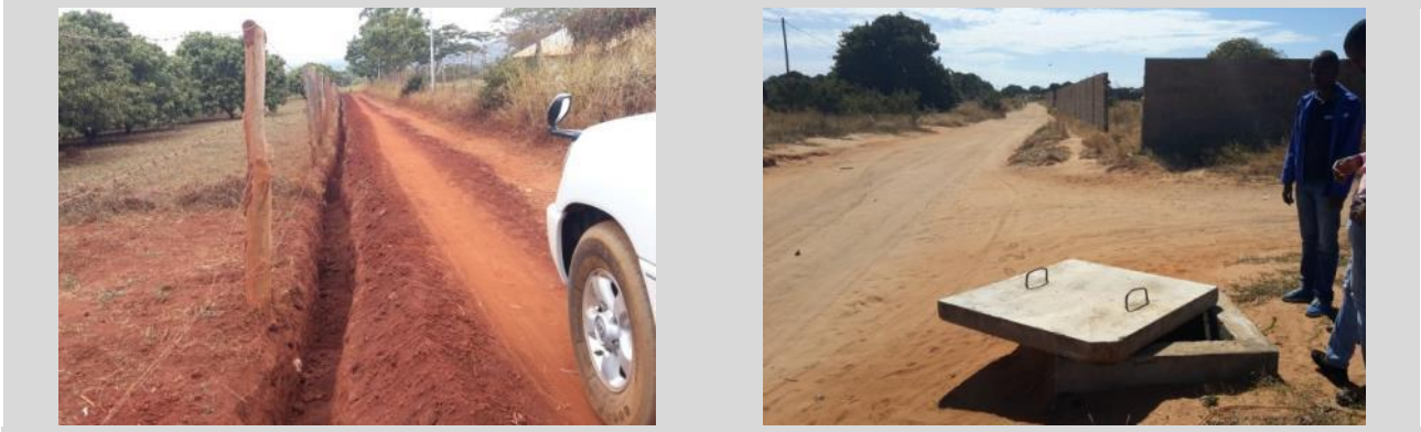
Figure 4-4: Distribution network expansion and maintenance, respectively in Chimoio (left) and Pemba (right)
