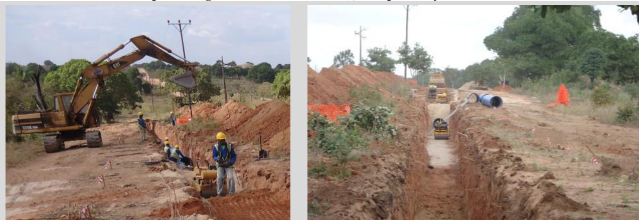
Figure 4-2: Civil works for a transmission main: Space required for safe operation of machines (top) and similar work in confined space using manual labour (bottom), Nampula City.
