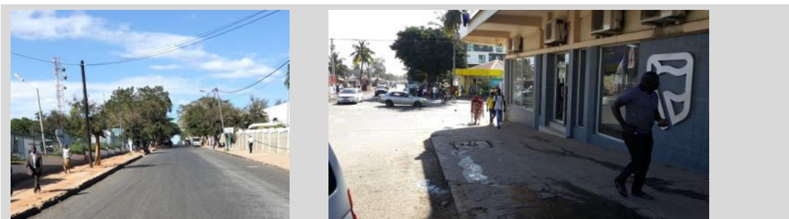
Figure 4-5: Paved areas and roads potentially to be degraded for pipes exchange in Pemba
