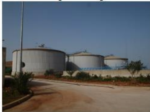
c. Anaerobic Digesters fo sludge treatment
