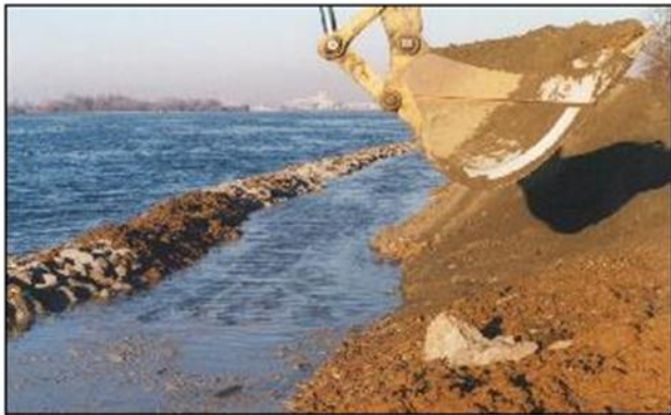
Ecological bank protection during construction (CNR – Rhône river 1998)
