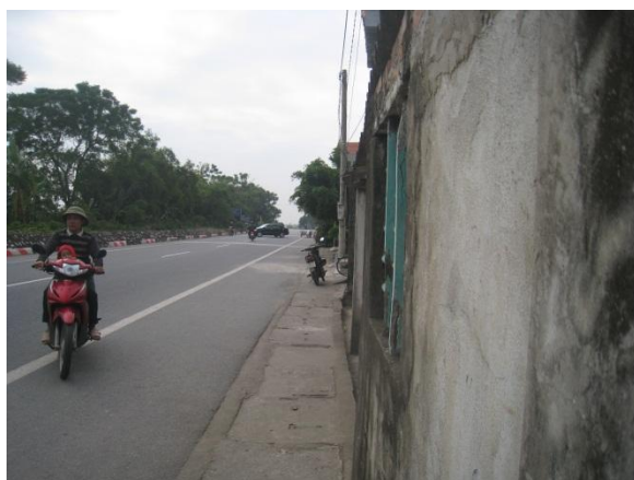
Starting point of project
