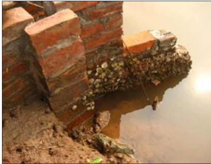
Figure 37 : Barnacles on the sluice gate near the rice paddy indicate constant presence of saline water
