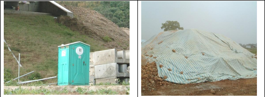
Figure 86: Latrines for Workers and Covered Construction Materials
