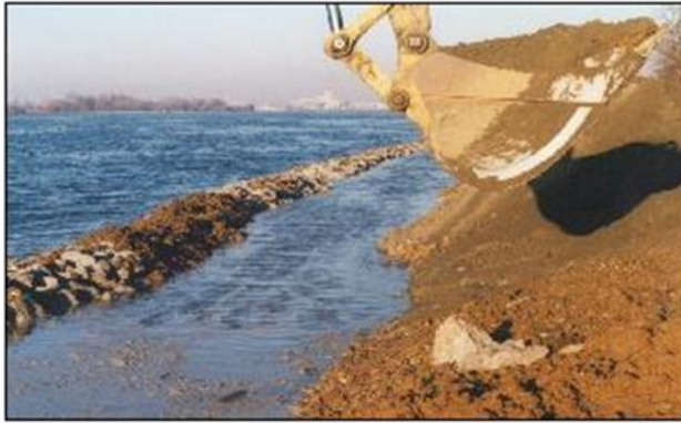
Ecological bank protection during construction (CNR – Rhône river 1998)
