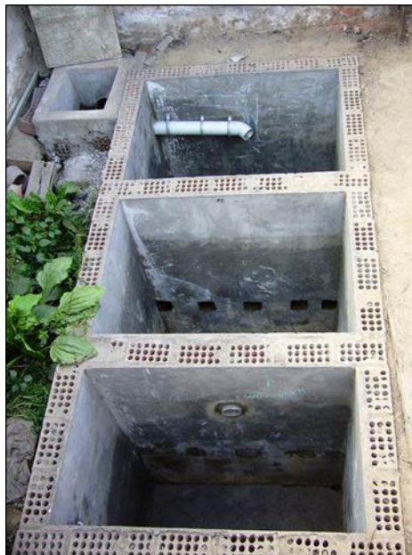
Figure 85: Picture of a rustic septic tank
