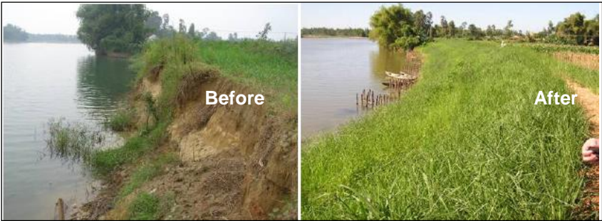
Figure 80: Vetiver River bank protection in Vietnam against flash flood
